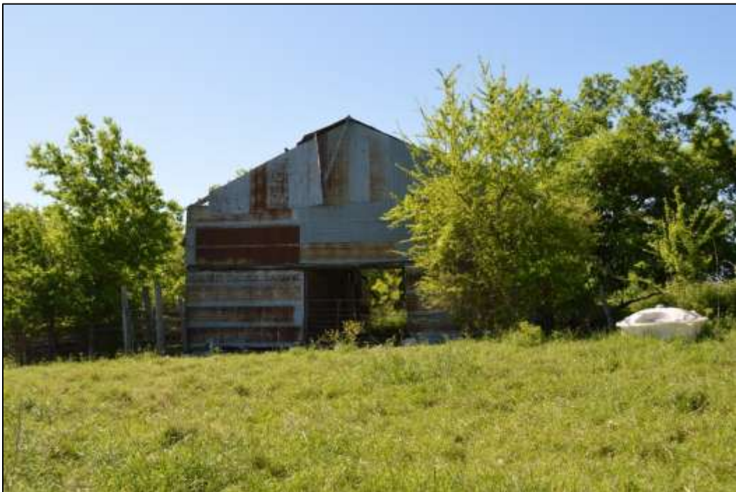
Figure 6-29. Resource 1C—View of Northern End of Hay and Livestock Barn (Facing South)
