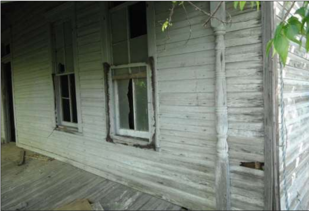
Figure 6-12. Resource 1A—Decorative Elements on Western Porch Façade (Facing Northeast)
