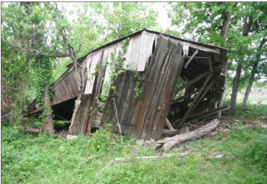
Figure 6-61. Resource 3B—View of the Barn (Facing West)
