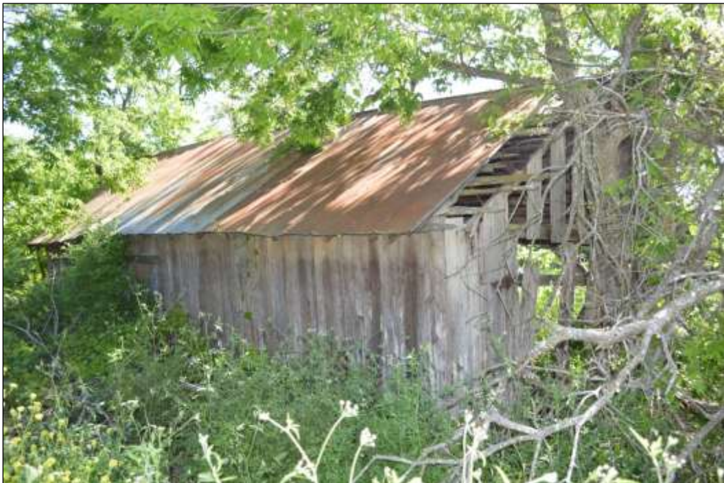
Figure 6-25. Resource 1B—View of Eastern Façade of Horse Barn (Facing Southwest)
