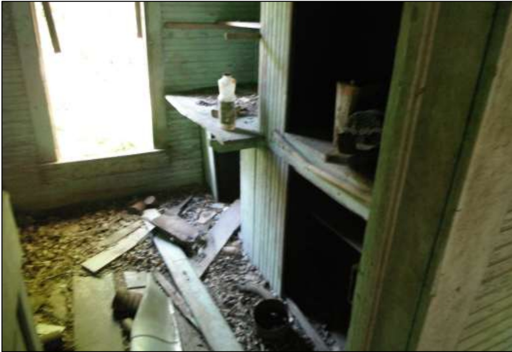
Figure 6-21. Resource 1A—View of Kitchen Pantry (Facing South)
