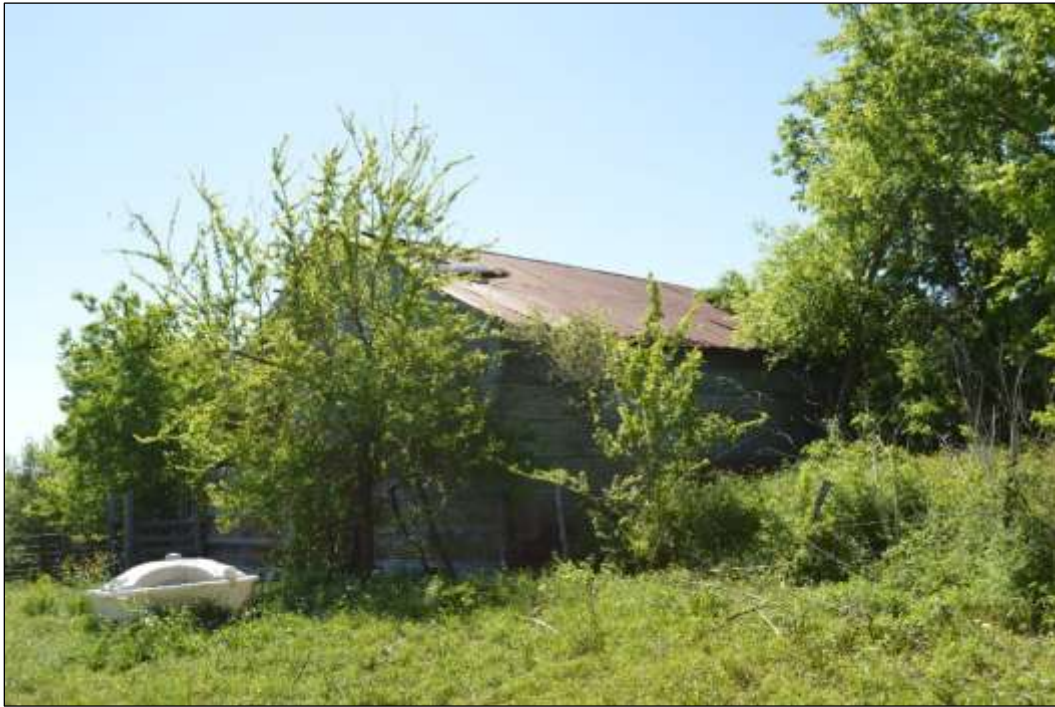
Figure 6-28. Resource 1C—View of Hay and Livestock Barn (Facing Southeast)
