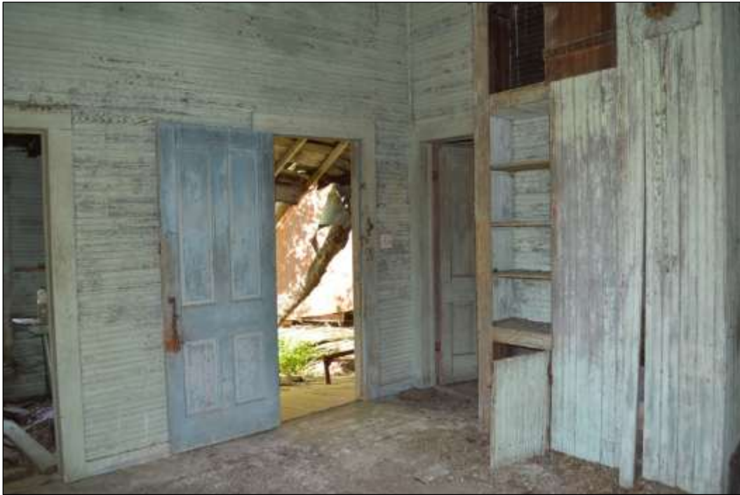
Figure 6-19. Resource 1A—View of Kitchen and Door Leading to Southern Porch (Facing Southwest)
