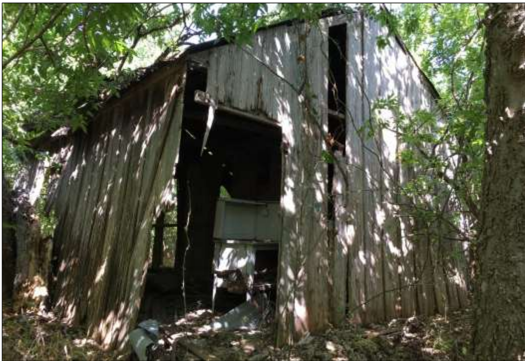
Figure 6-76. Resource 4—View of Rear Façade of Garage (Facing West)
