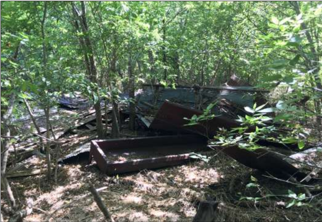
Figure 6-80. Collapsed Outbuilding West of Barn on Site 41TV2522 (Facing North)
