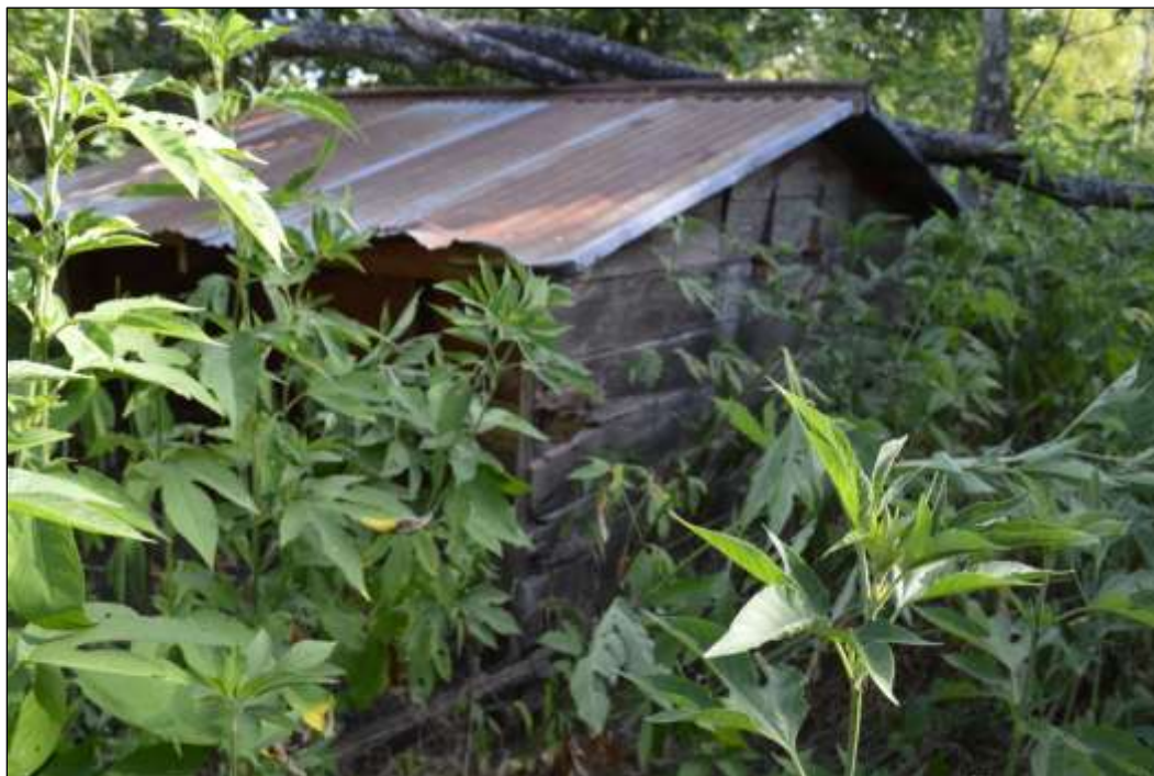
Figure 6-34. Resource 1D—View of Livestock Feeder (Facing Northwest)
