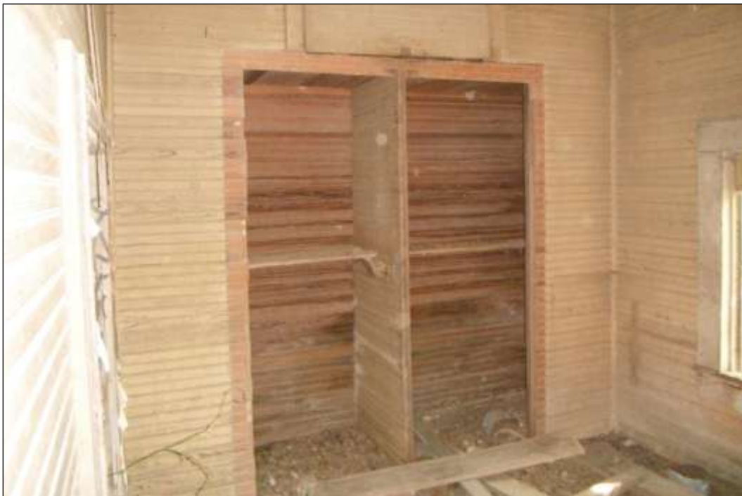
Figure 6-18. Resource 1A—View of Child’s Bedroom (Facing Northeast)
