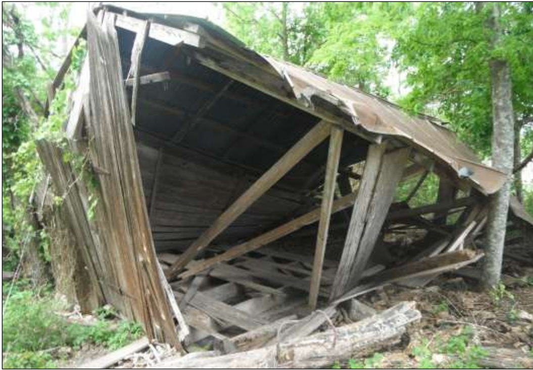
Figure 6-62. Resource 3B—View of the Barn (Facing Southwest)
