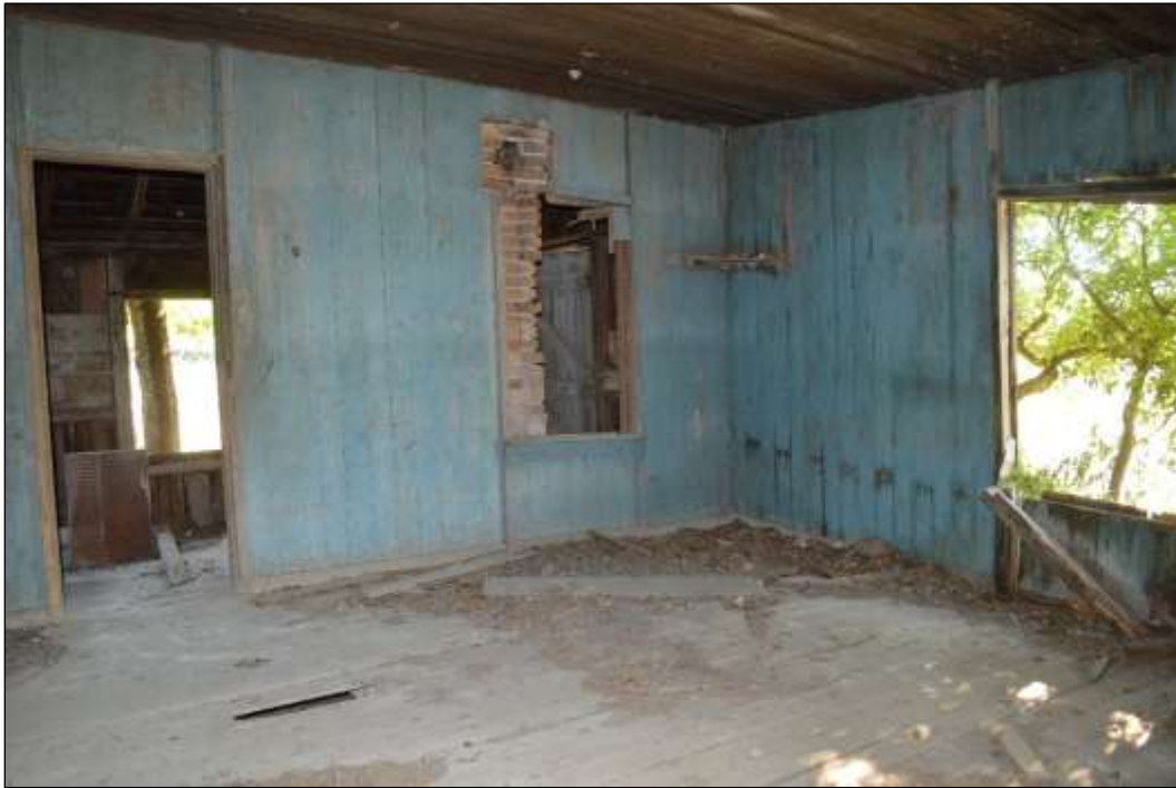
Figure 6-47. Resource 2—View of Southeastern Room (Front Parlor) (Facing Northeast)
