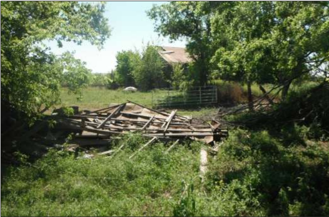
Figure 6-35. View of Debris Pile (Collapsed Former Outbuilding) on Site 41TV2518 (note Resource 1D in background) (Facing Southeast)
