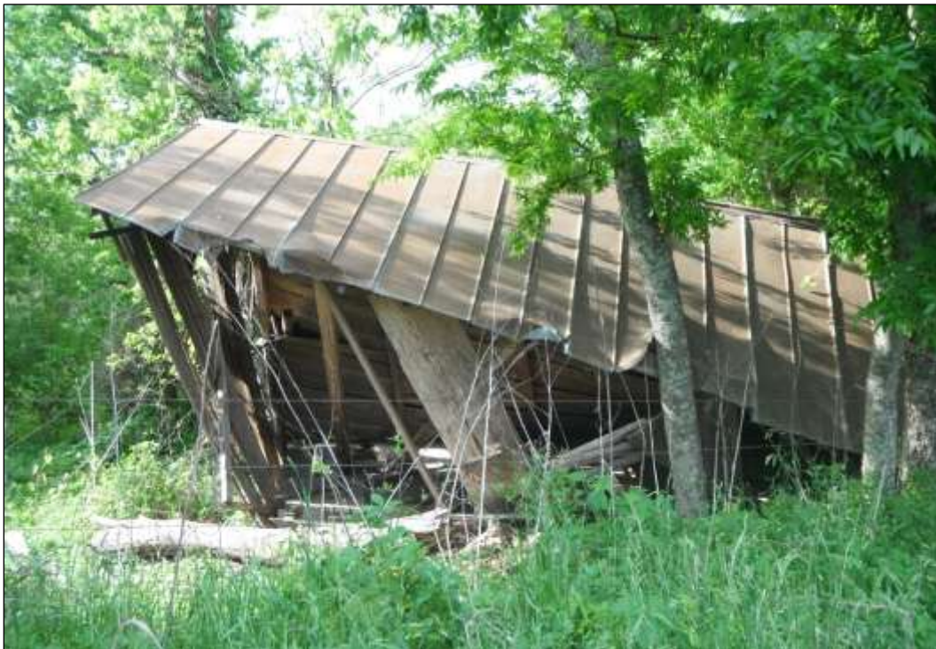
Figure 6-63. Resource 3B—View of the Barn (Facing South)
