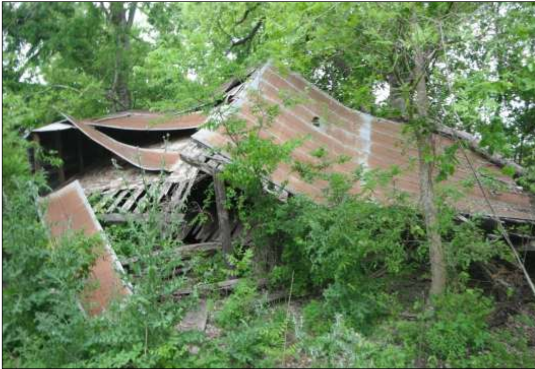
Figure 6-60. Resource 3A—View of the House (Facing West)
