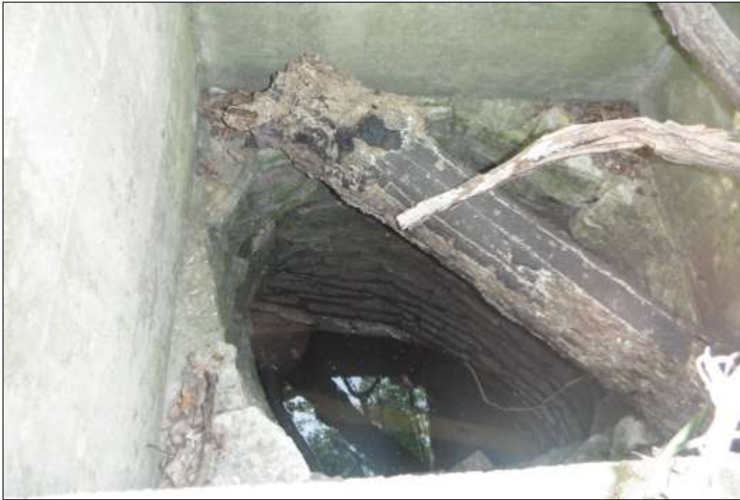
Figure 6-65. Interior of Limestone Well (Facing East)
