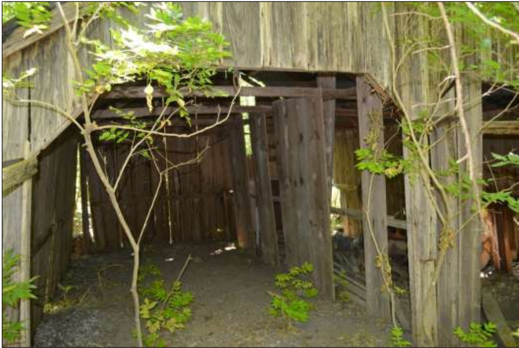
Figure 6-77. Resource 4—Interior of Garage (Facing Northeast)
