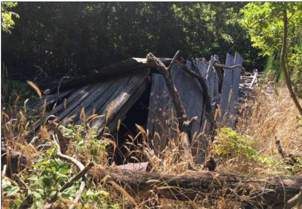
Figure 6-78. View of Collapsed Barn on Site 41TV2522 (Facing South)
