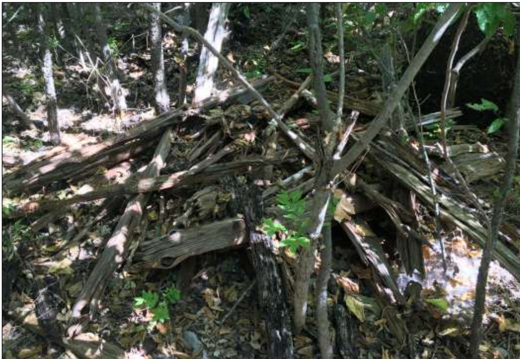
Figure 6-79. Collapsed Outbuilding Northeast of Barn on Site 41TV2522 (Facing North)
