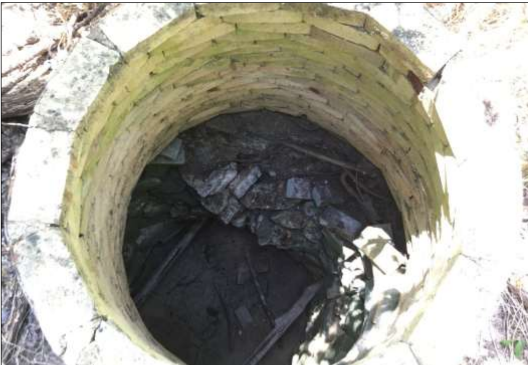
Figure 6-72. Interior of Stacked Limestone Well on Site 41TV2521
