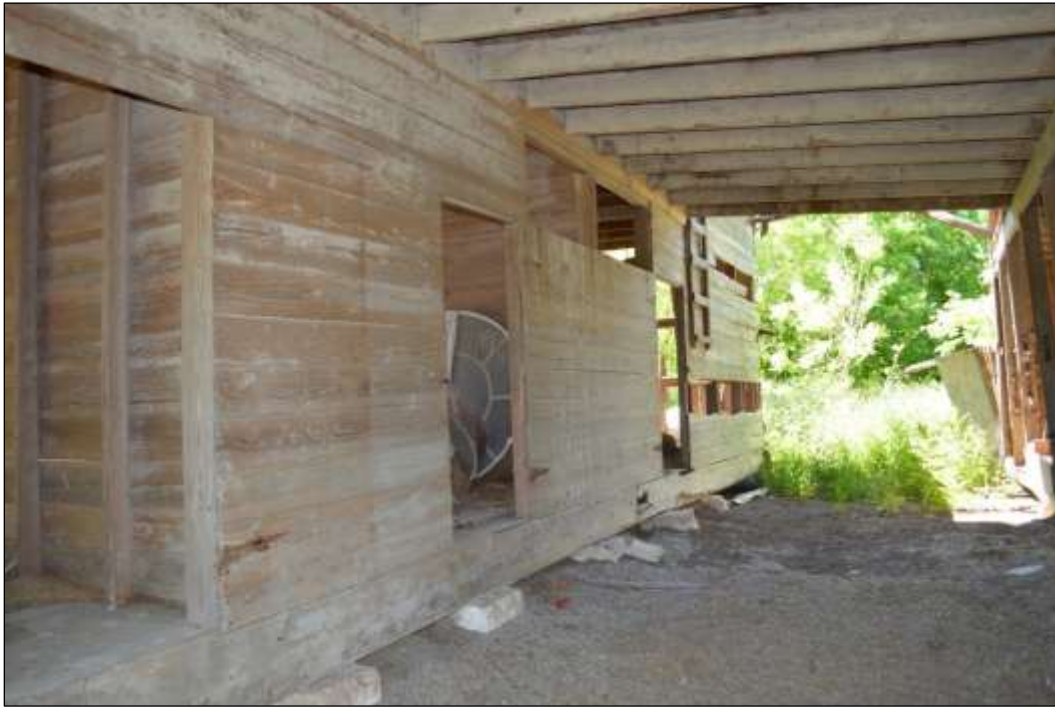
Figure 6-32. Resource 1C—Enclosed Bays along Eastern Side of Barn Interior (Facing Southeast)
