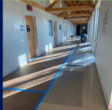
Justice Center Sewer Line Project
