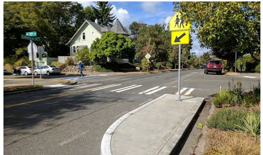
Example of a paved intersection bulb out.
