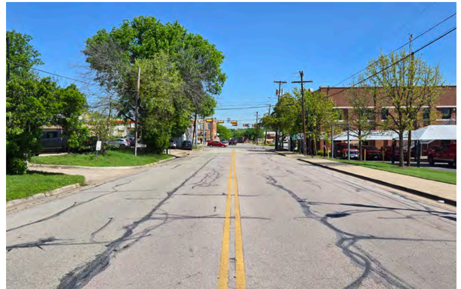
Railroad Avenue and Hall Street viewing north toward Pecan Avenue.
