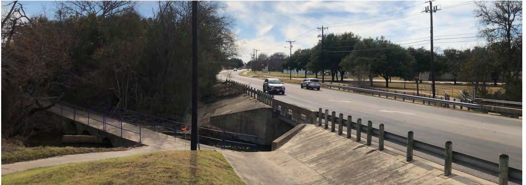
Looking south at Railroad Avenue and Gilleland Creek.
