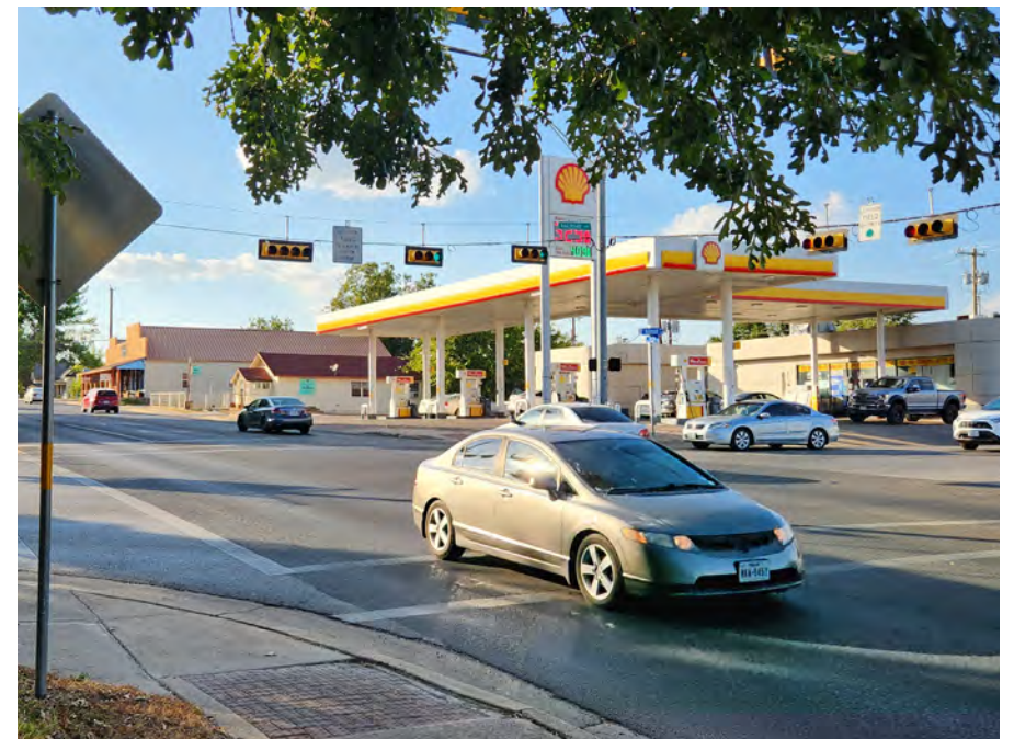
Pedestrian crossing facilities meet minimum standards.
