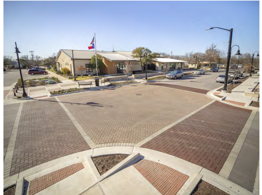
Colored Thermoplastics application at an intersection.
