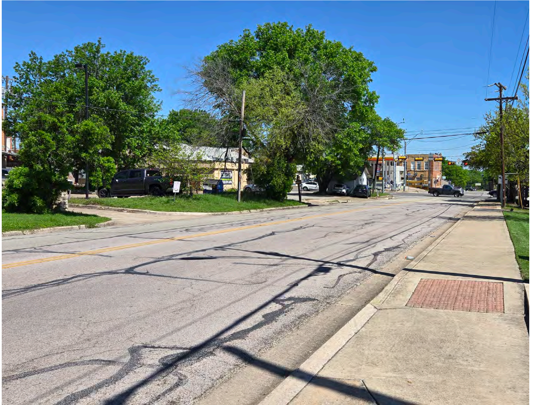
View of Railroad Avenue at Hall Street looking North.
