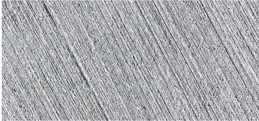
Broom finish concrete
