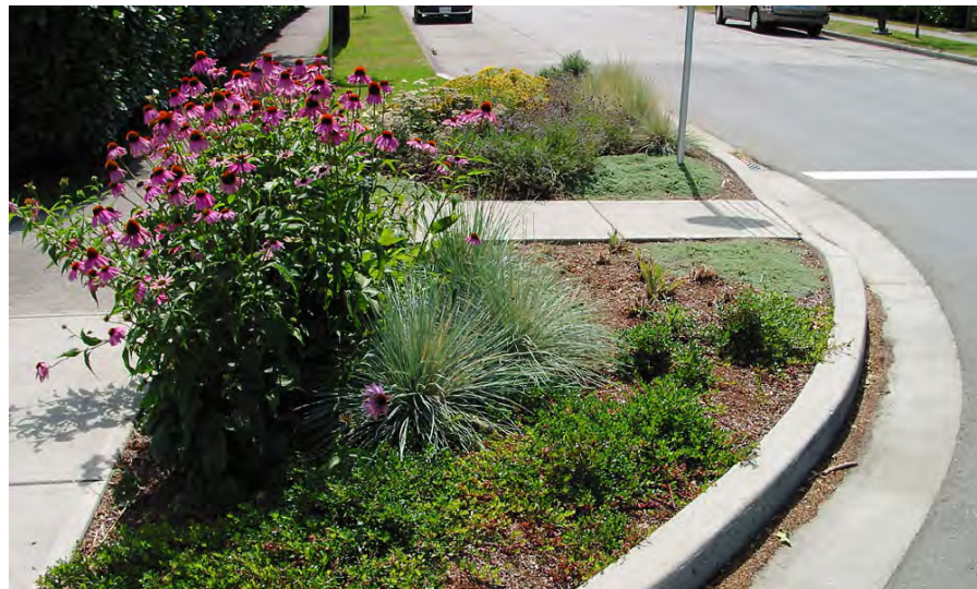
Example of a planted intersection bulb out.
