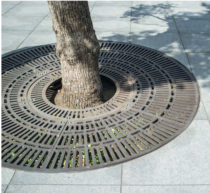
Tree grates with removeable center rings allow tree trunks to grow.
