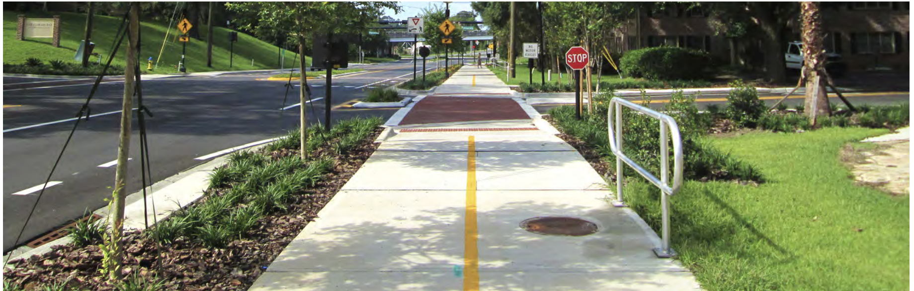
Example of shared-use path separated from roadway with ornamental plantings.
