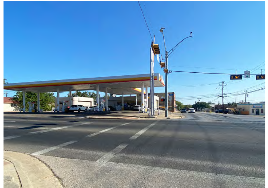
Existing view from south corner of Pecan Street and Railroad Avenue viewing north.
