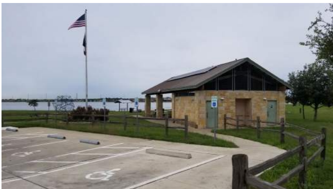
PICTURE 03 | LAKE PFLUGERVILLE - RESTROOM
