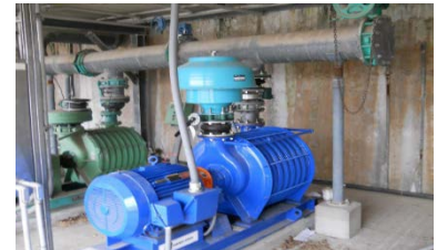
Central Wastewater Treatment Plant Improvements
