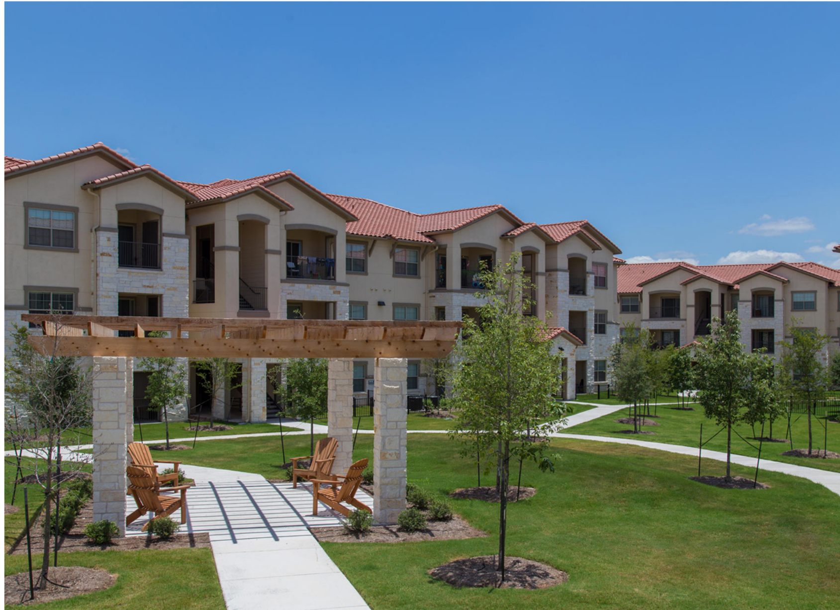
TYPICAL 3 STORY RESIDENTIAL BUILDING Stucco and limestone exterior materials with clay tile roof
