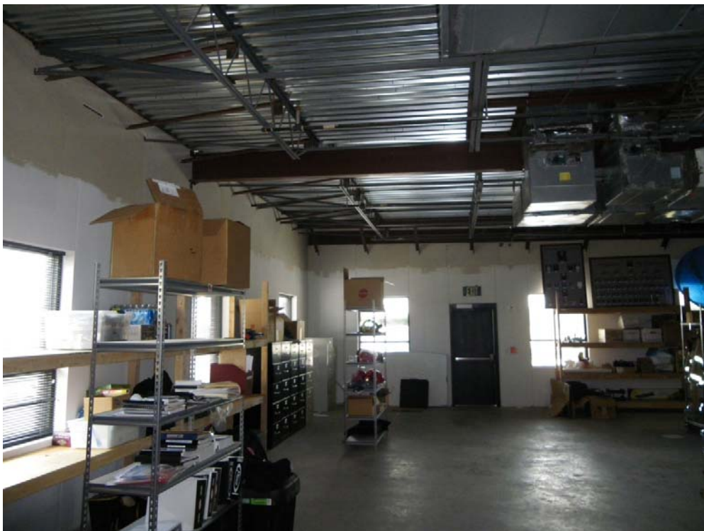
12. Travis County ESD No. 2 – 2 nd Floor Facility
