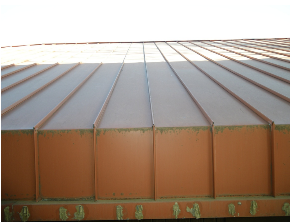
6. Existing standing seam roof – Building 200: Typical conditions observed on all buildings
