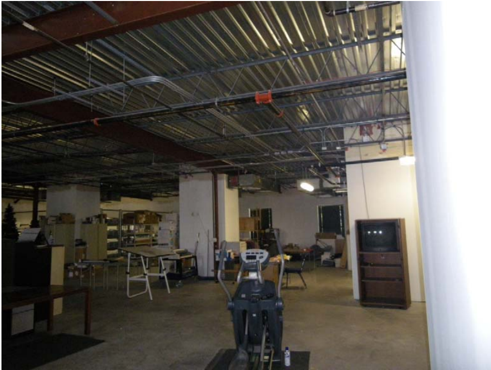
11. Travis County ESD No. 2 – 2 nd Floor Facility
