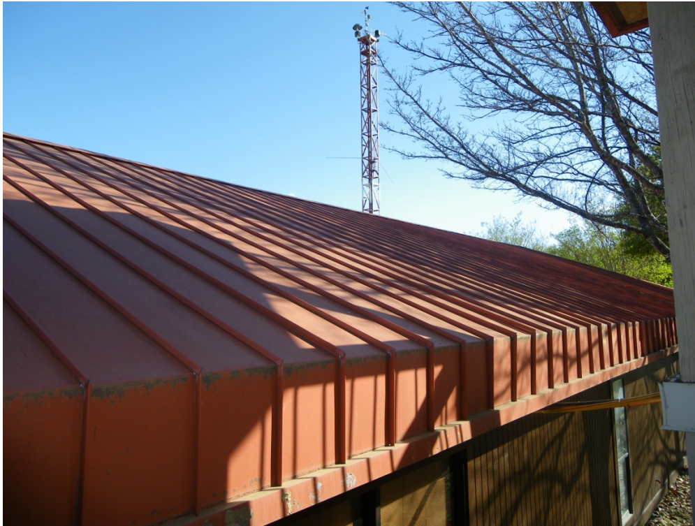
7. Existing standing seam roof – Building 200: Typical conditions observed on all buildings
