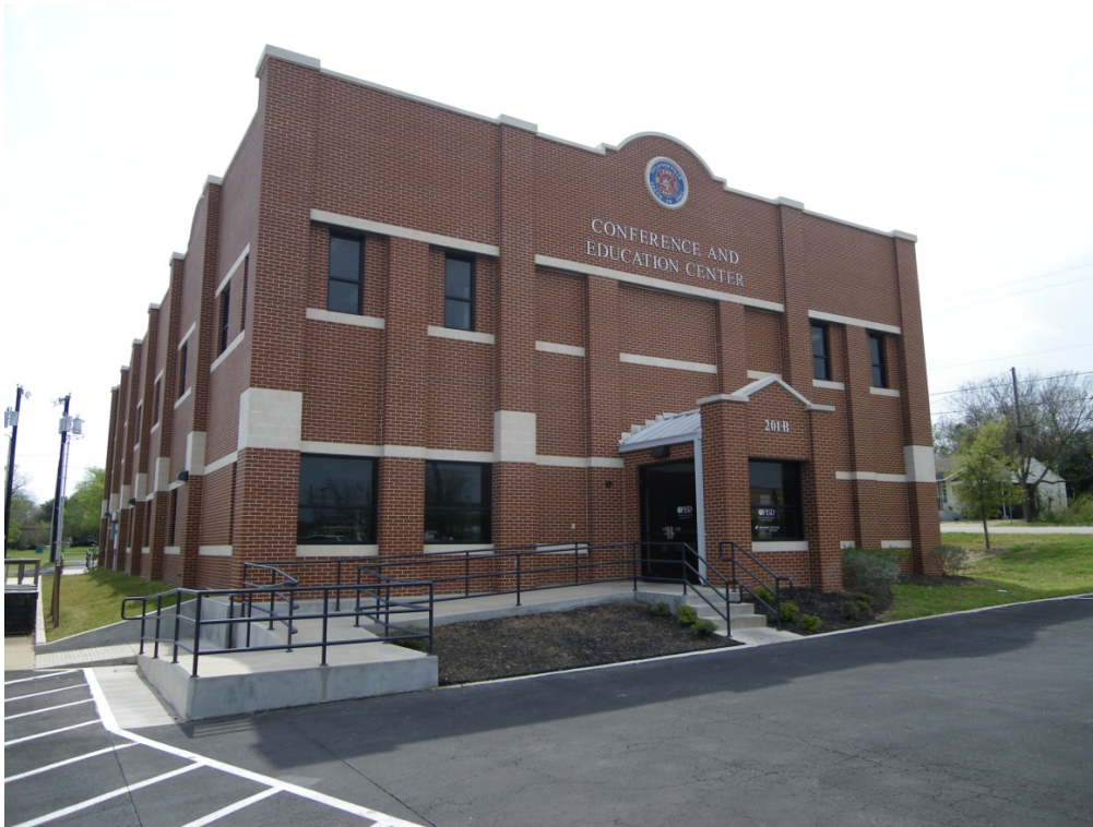
9. Travis County ESD No. 2 – Conference and Education Center
