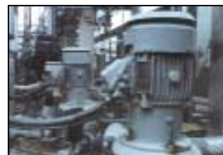
Duty Master XT Vertical Motors drive in-line process pumps in petroleum refining operation.
