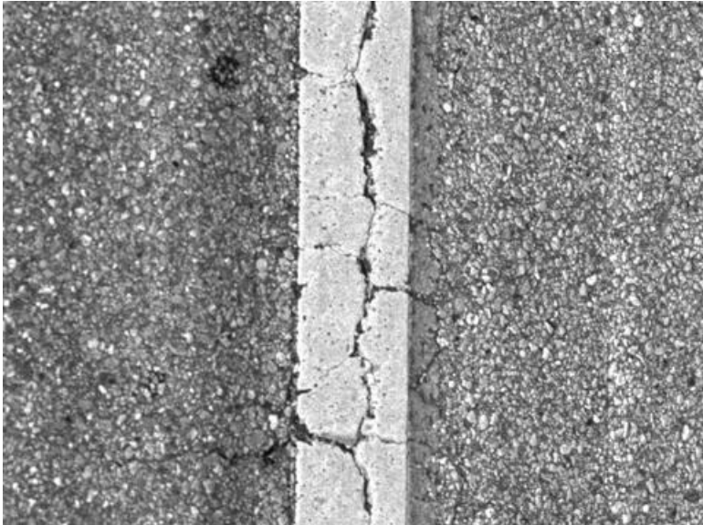
Pavement image captured with the 4K LRIS
