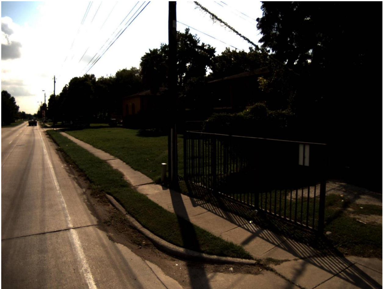
Sample image of curb and gutter collected with MAC system
