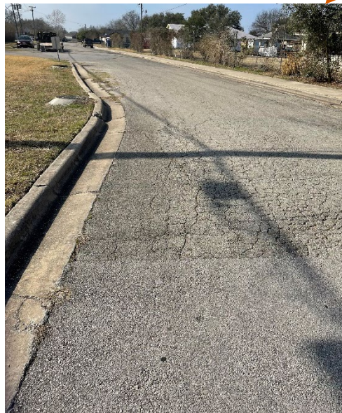
Alligator Cracks
