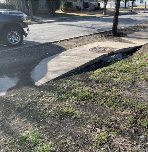
Vertical Movements on Sidewalk
