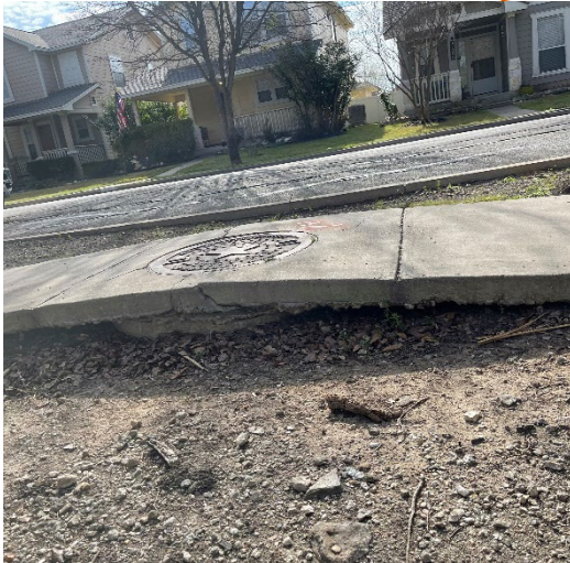
Vertical Movements on Sidewalk
