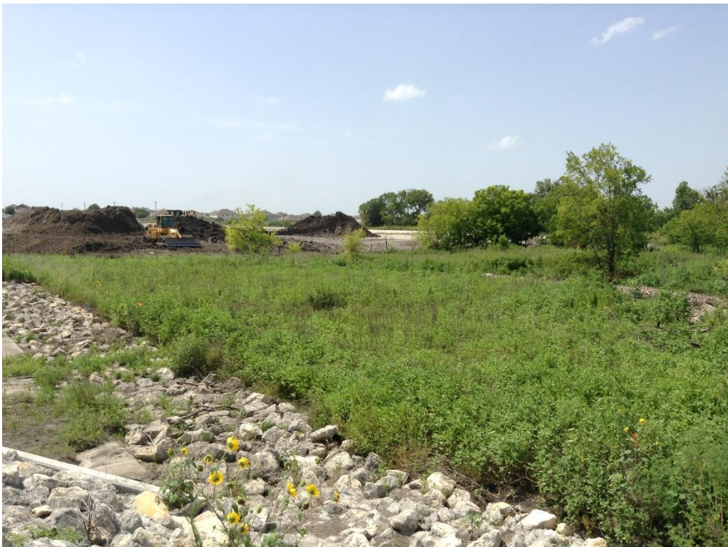
Photo 4: North side of culvert crossing at Town Center Drive, facing north. Construction of new houses on western boundary.
