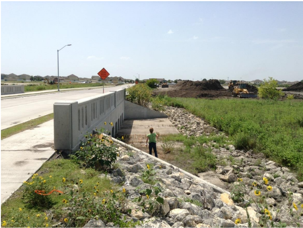
Photo 3: North side of culvert crossing at Town Center Drive, facing west. Tributary does not contain water at this location.
