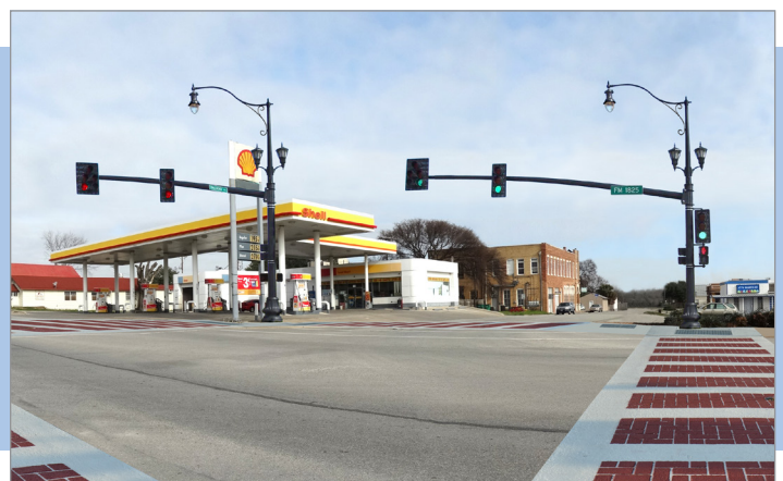
Anticipated conditions at Pecan Street and Railroad Avenue
