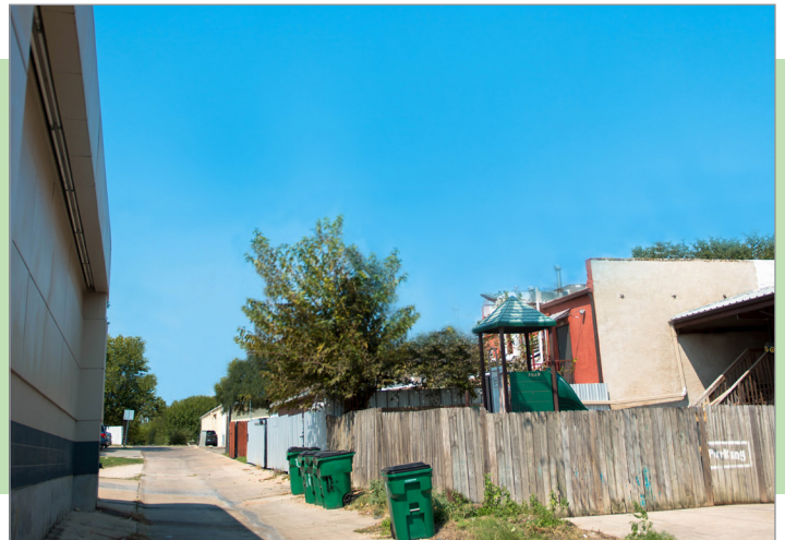
Anticipated conditions at Alley at N. Railroad Avenue after the overhead utilities are placed underground
