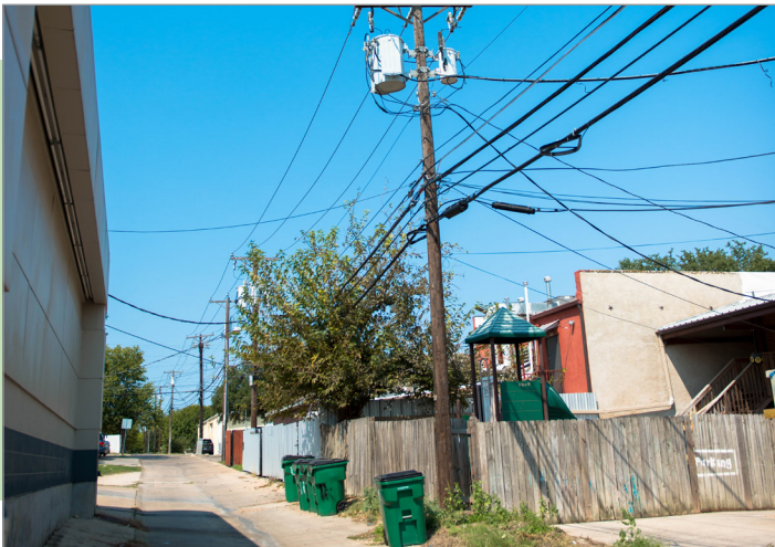
Existing conditions at Alley at N. Railroad Avenue
