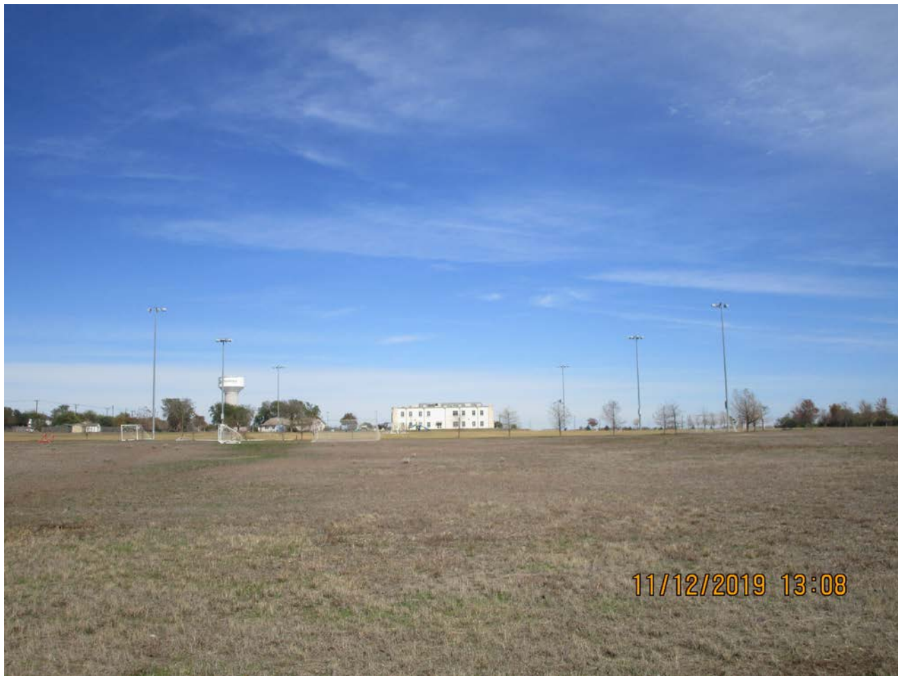
Photo taken from Black Locust Dr, showing the existing athletic field lighting, light fixtures.
