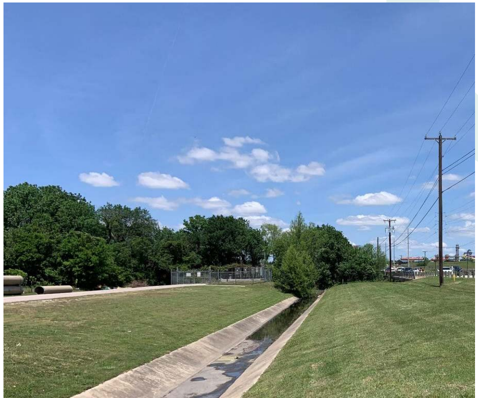
Figure 3-16: Wastewater Lift Station Along FM 685
