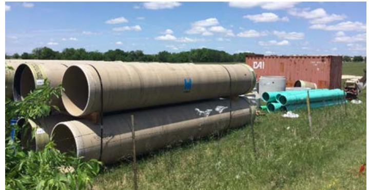
Figure 3-18: Drainage Culverts Prepared for Installation Along FM 685
