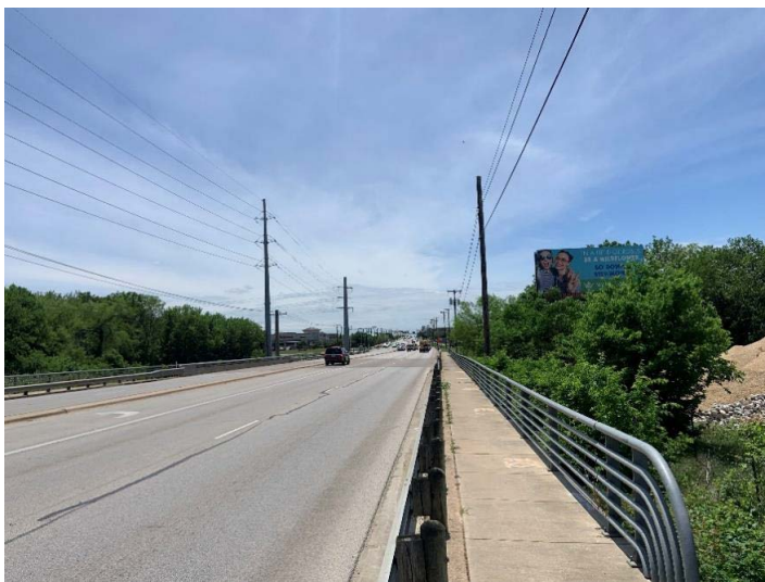
Figure 3-4: Bridge Crossing Wilbarger Creek
