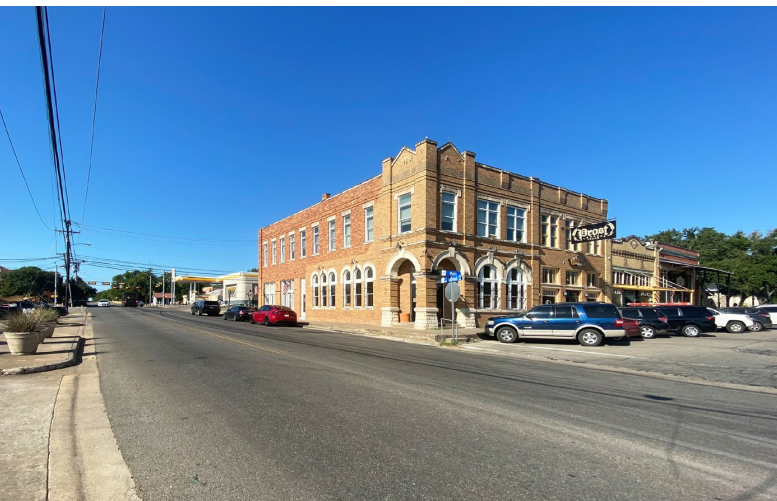
Existing view from northeast corner of Main Street and Railroad Avenue.
