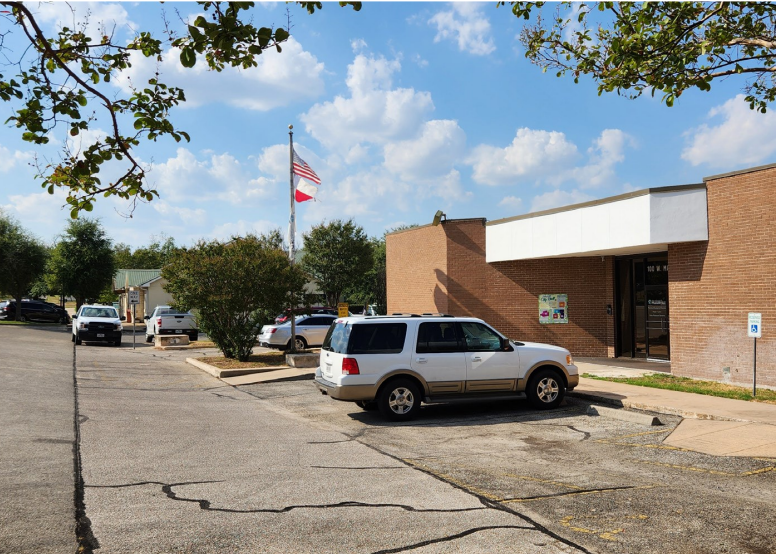
Existing view from southeast entrance of the City office.
