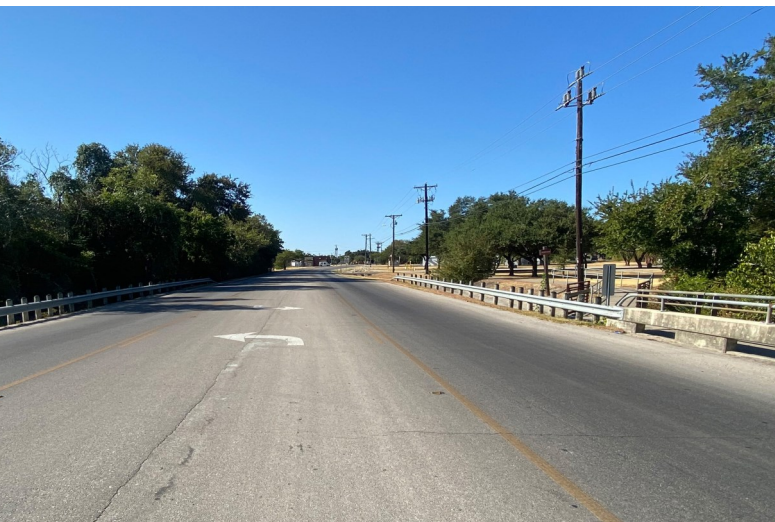
Existing view traveling south on Railroad Avenue, passing Gilleland Creek.
