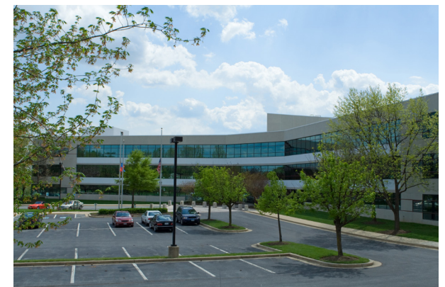
Parking lot outside of an office building
