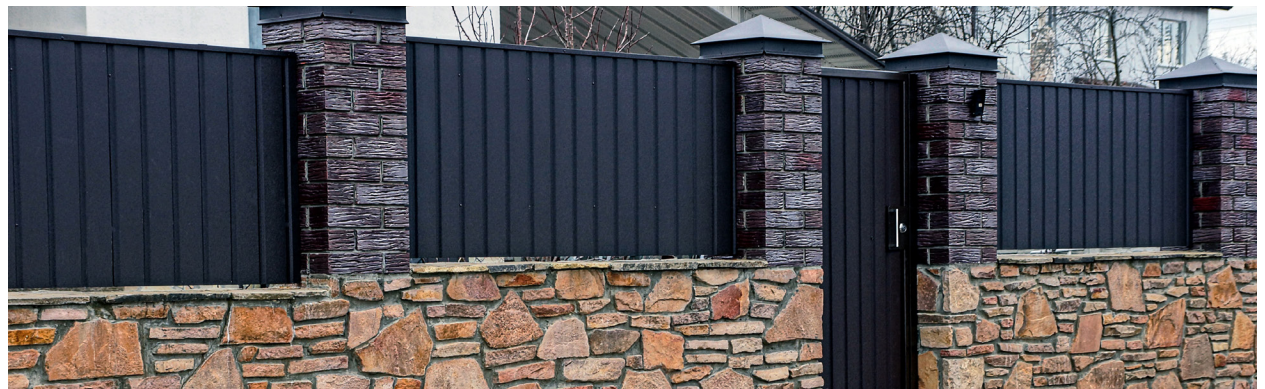
Screening Wall Metal Masonry
