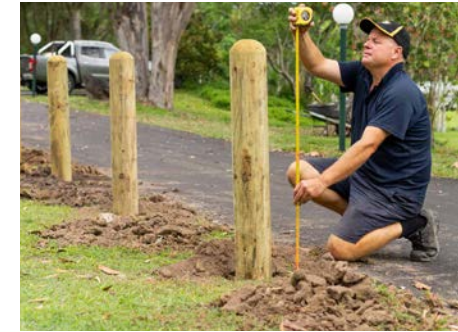
Wood Bollard - Trails: 6"Ø Pressure treated wood bollard w/ 3" radius top (Pflugerville Parks & Rec Department Standard Furnishing)
