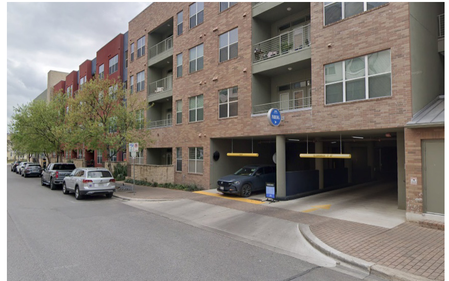
An example of a curb cut at a structured parking entrance that ramps up to the level of the sidewalk so that the sidewalk and its treatment remain consistent across the driveway.
