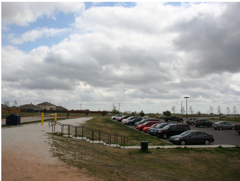
Variable materials for trail and parking and the lack of a containment edge
