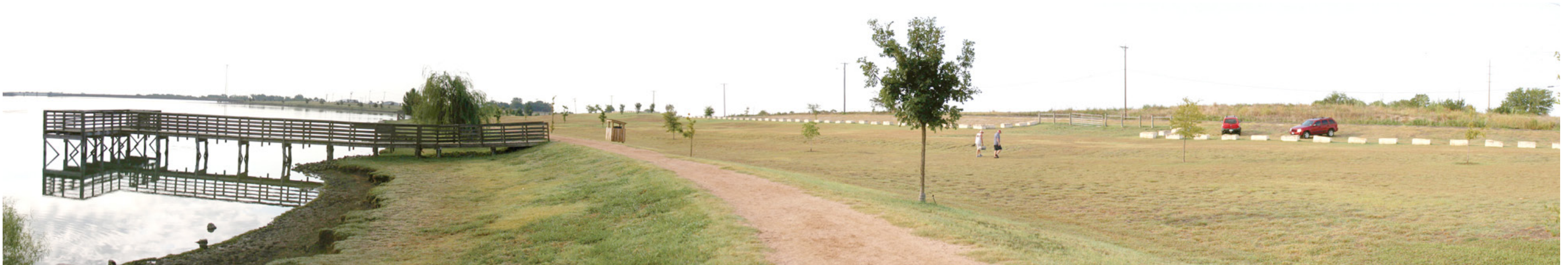
Before - Existing Fishing Pier and Varying Width Decomposed Granite Trail
