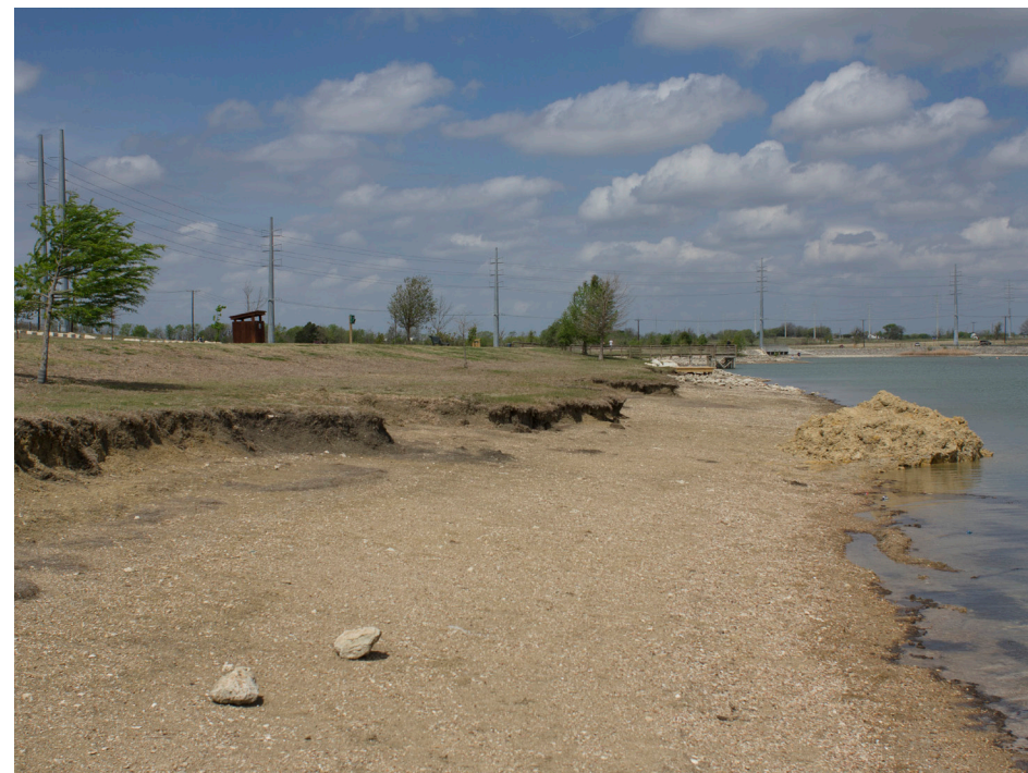
Significant erosion and receding shoreline is present at the south bank
