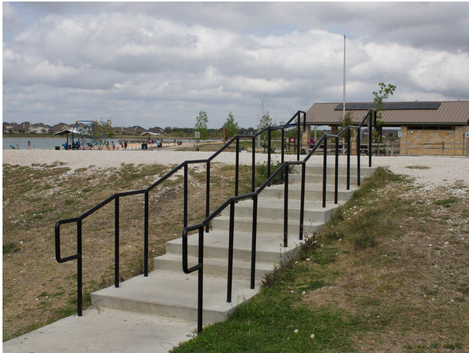
Limited accessible routes within activity areas and from parking
