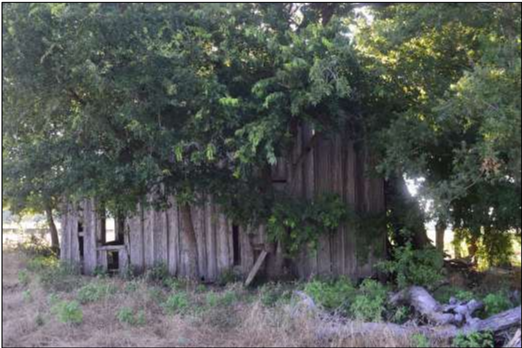
01. West façade of house
