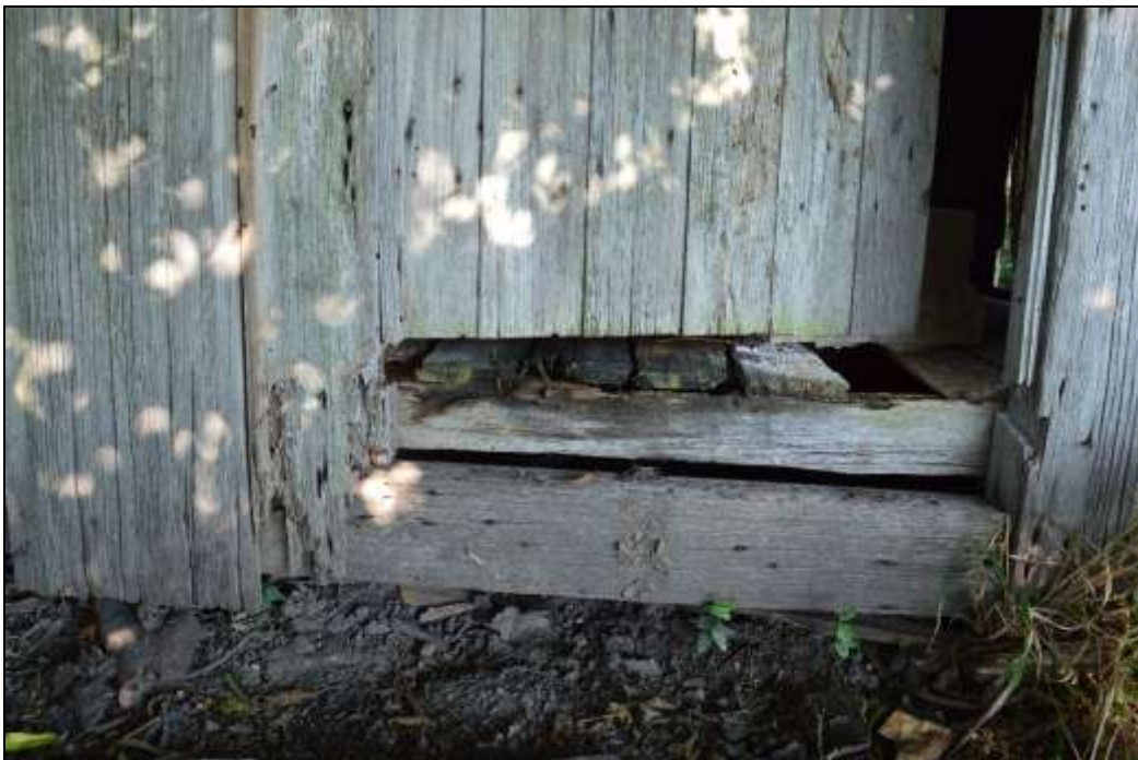
16. Floor construction below kitchen door on east façade of house
