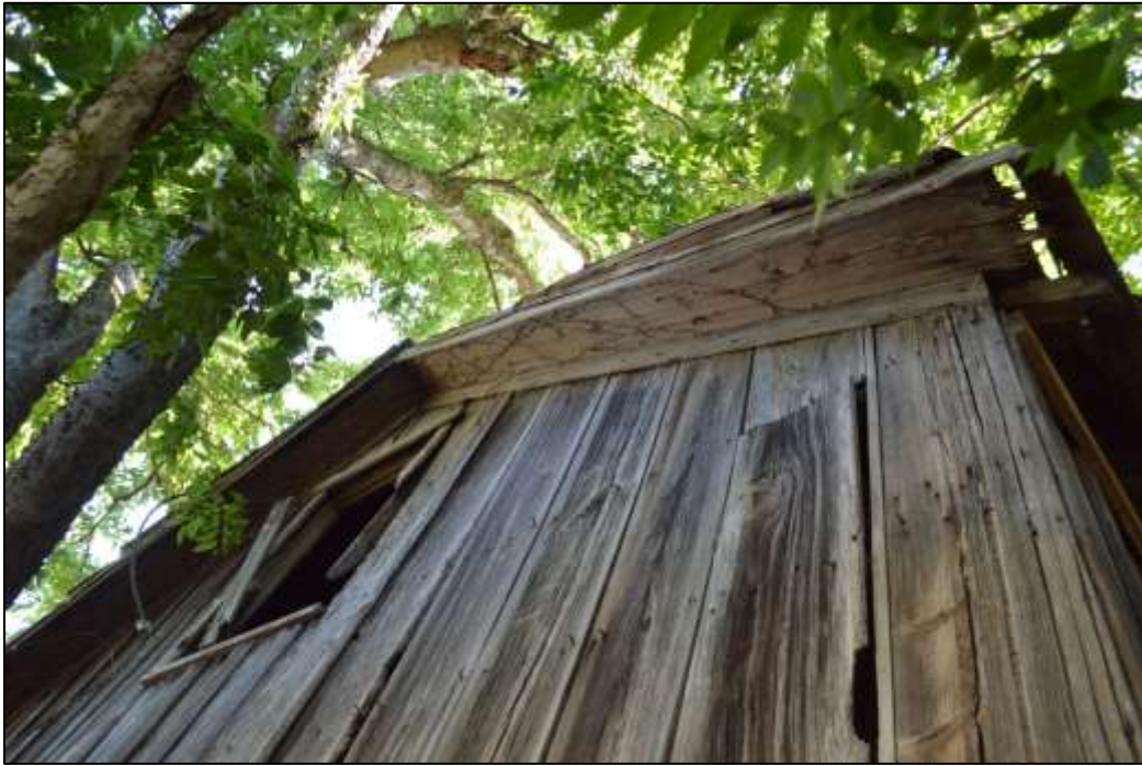
31. Exterior roofing, lightning grounding rod, and cornice/eave details
