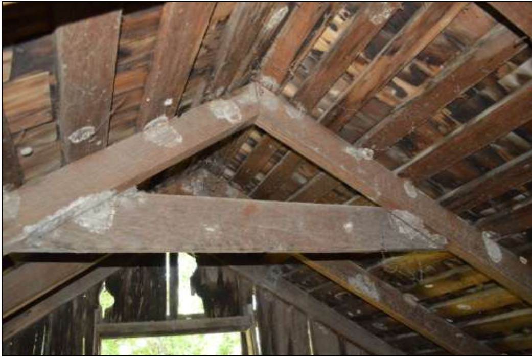
39. Roofing in loft showing rafters
