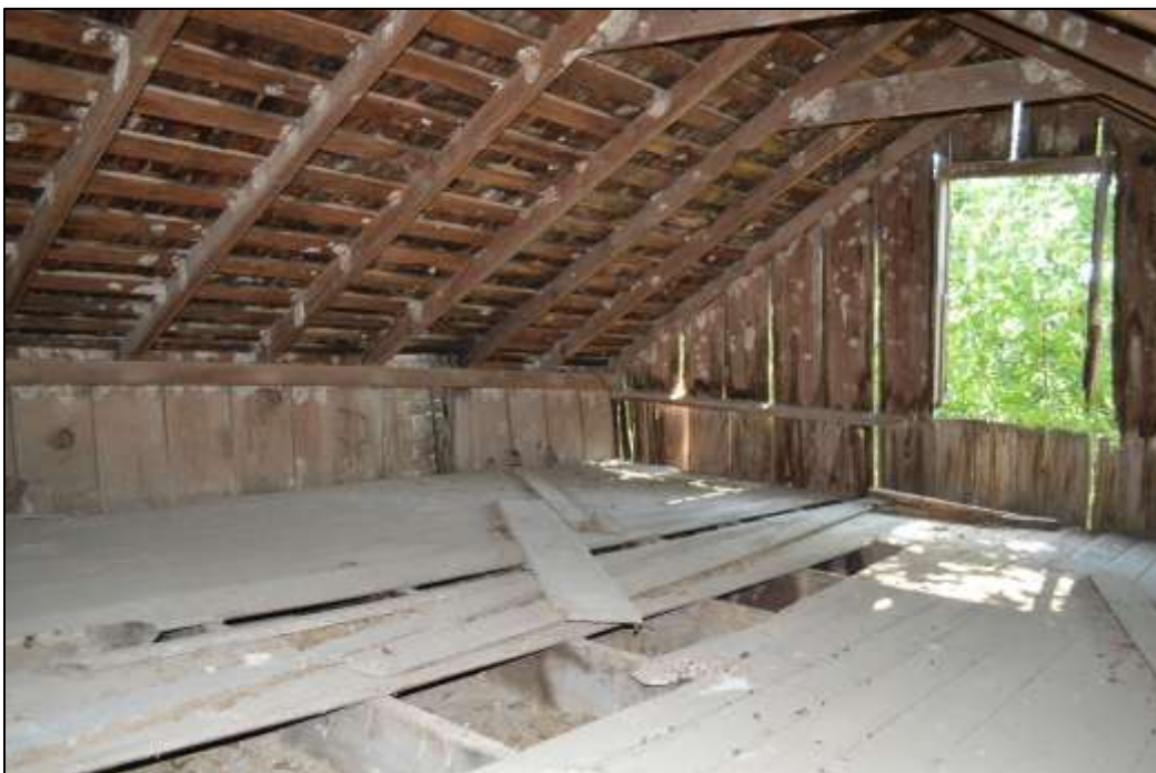
68. Interior of loft
