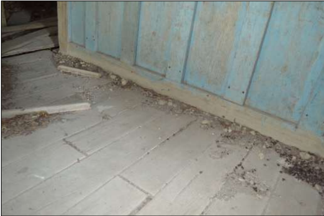
45. Interior flooring, baseboards, and walls in southeast room
