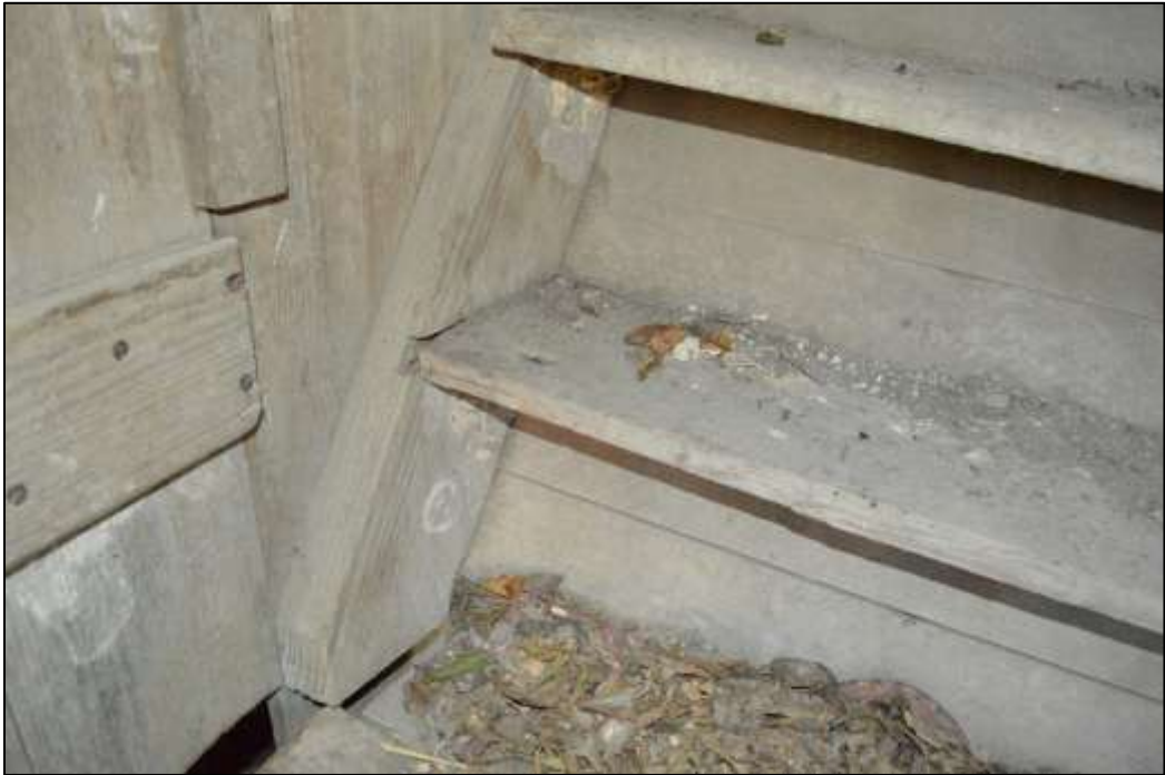
41. Detail of stairs
