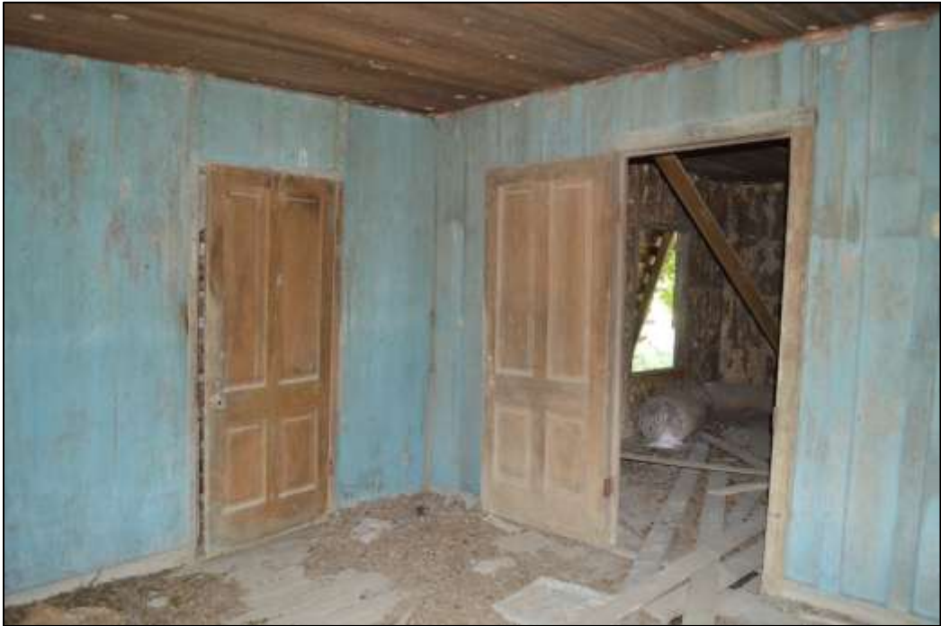
65. Interior of southeast room
