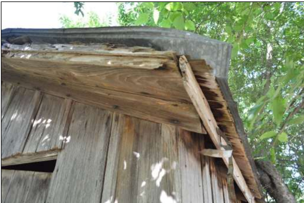
34. Roof cornice at northeast corner of house
