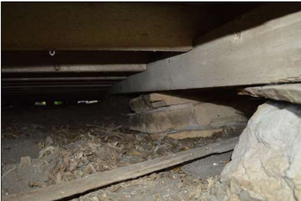
12. Pier under the north wing
