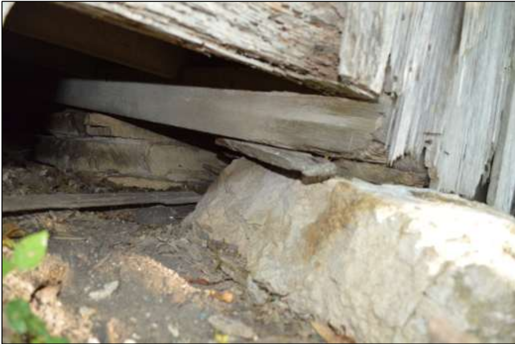
11. Pier under the north wing
