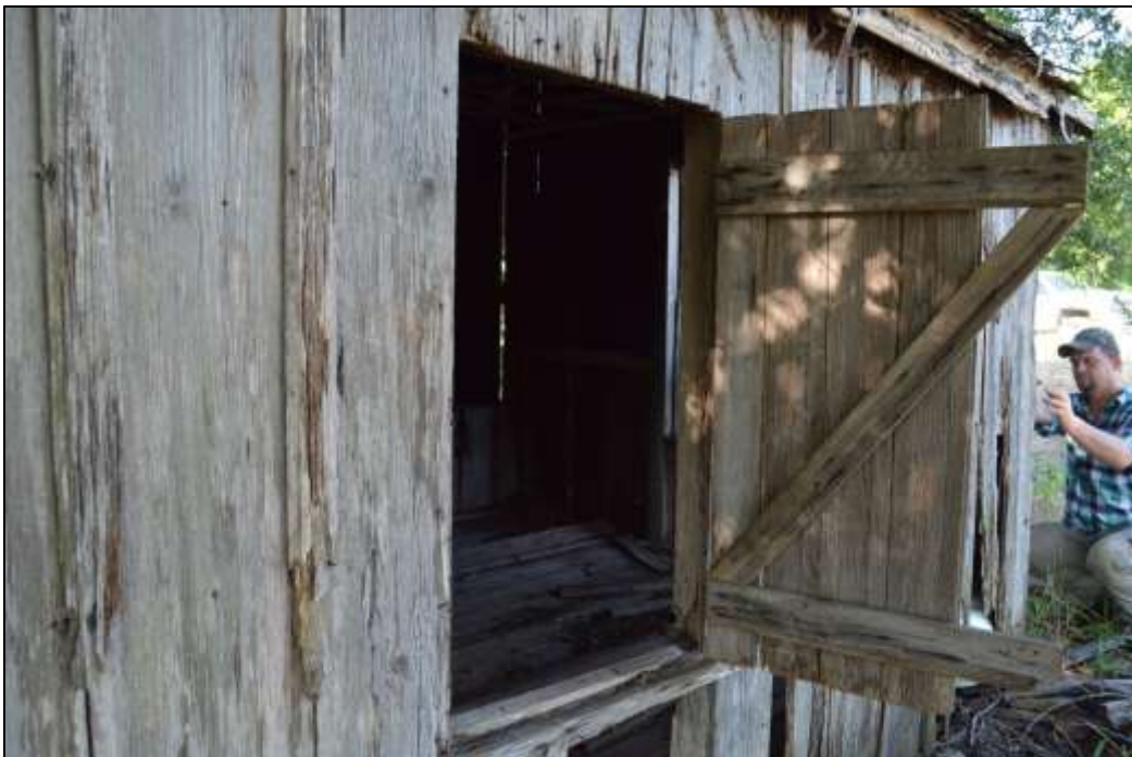
20. Exterior window on the west side of the north façade
