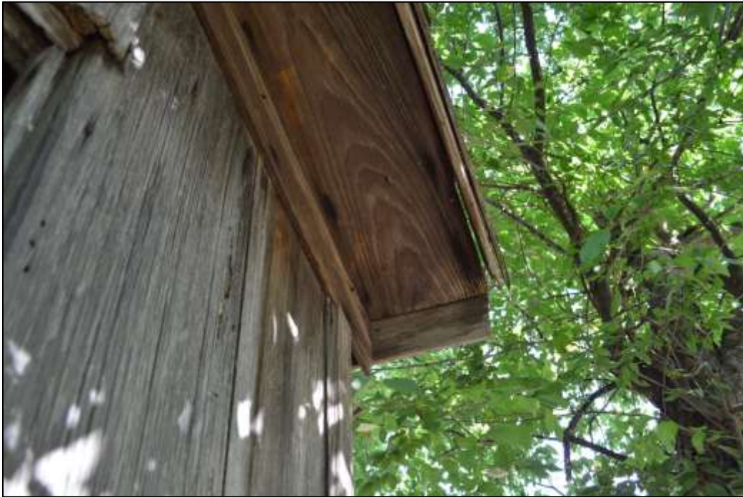
33. Roof cornice and eave at northeast corner of house
