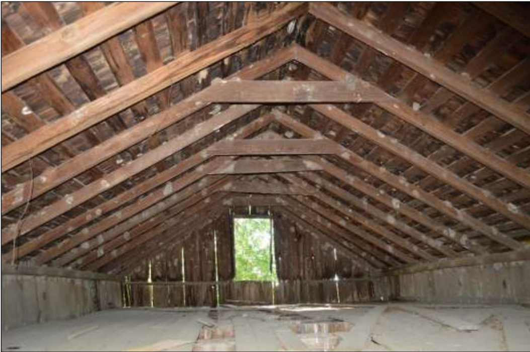
Figure 13. View of Second (1/2-) Story Sleeping Loft (Facing East)
