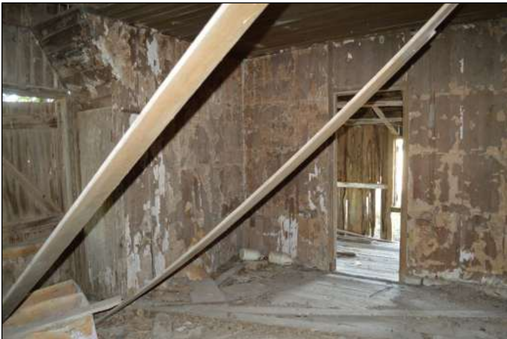
52. Interior overview of southwest room
