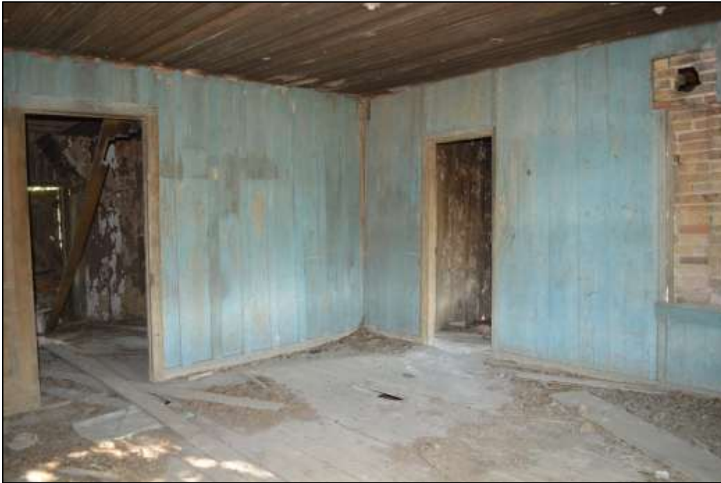
55. Interior overview of southeast room
