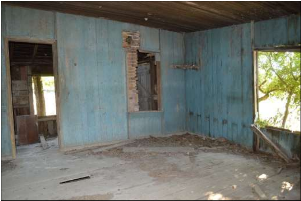
54. Interior overview of southeast room
