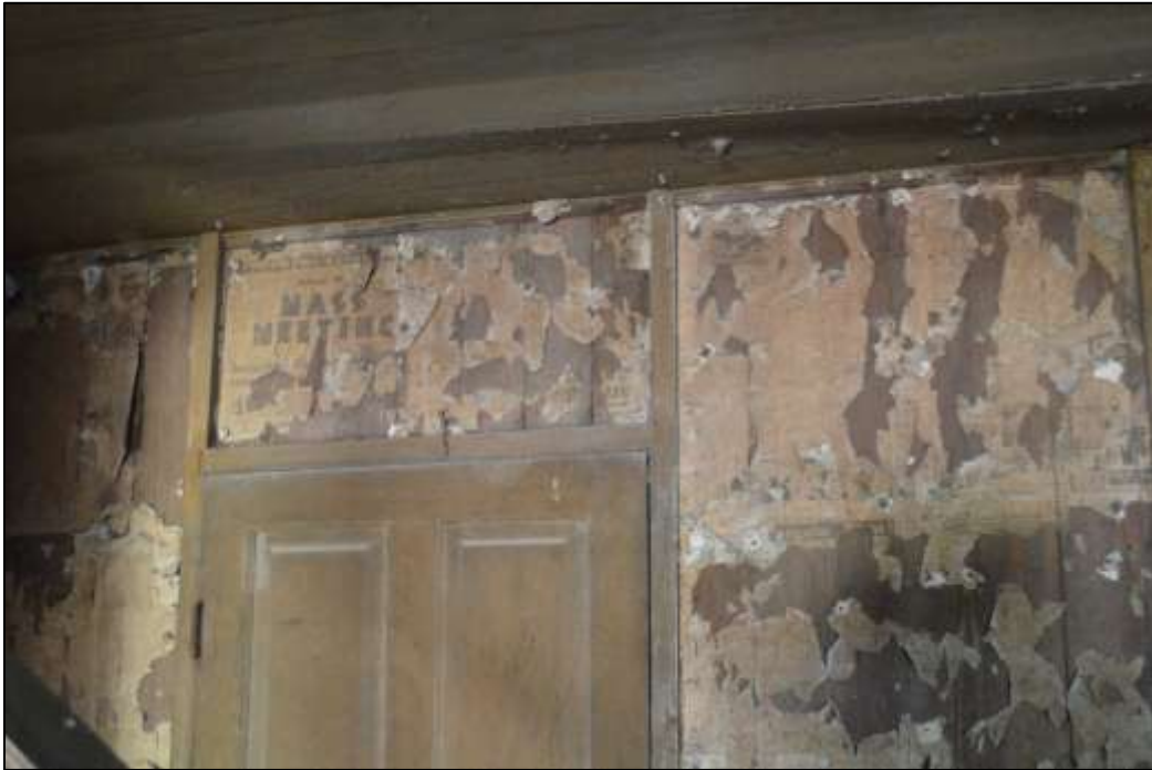
51. Interior walls and roofing in southwest room showing newspaper on walls
