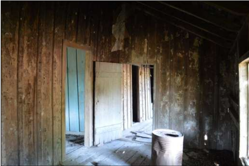
59. Interior overview of northeast room (kitchen)
