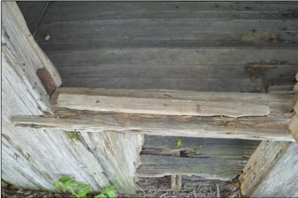
21. Window opening showing sills on north façade of house
