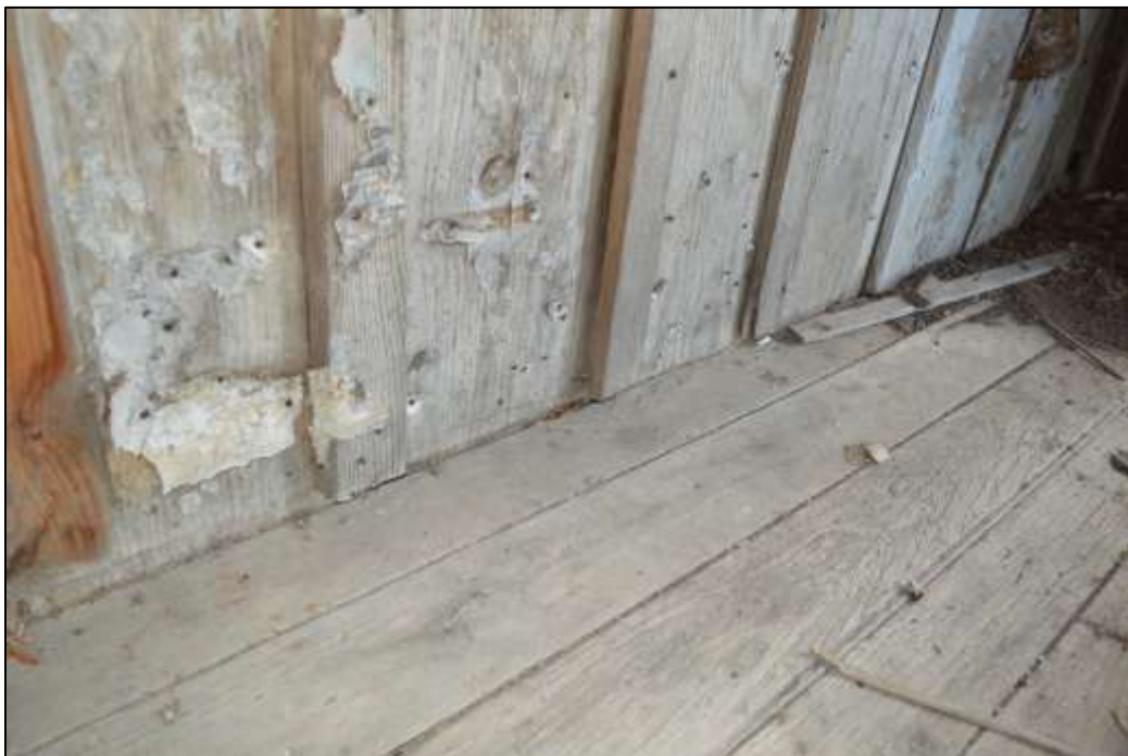
44. Interior flooring and walls in northwest room
