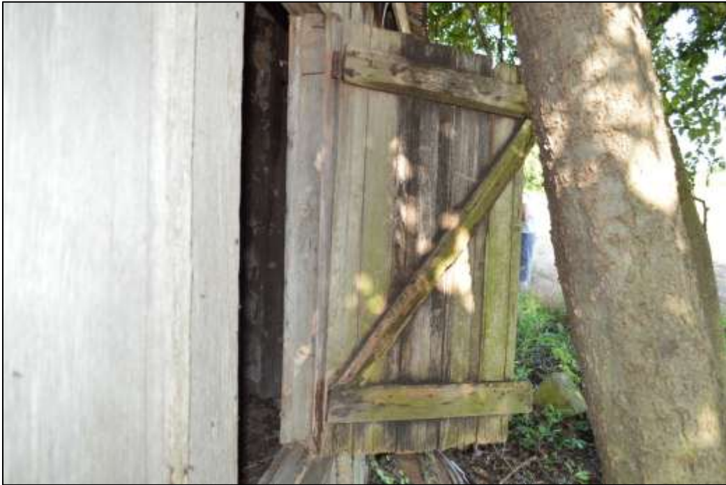
19. Wooden window shutter on the east side of the north façade
