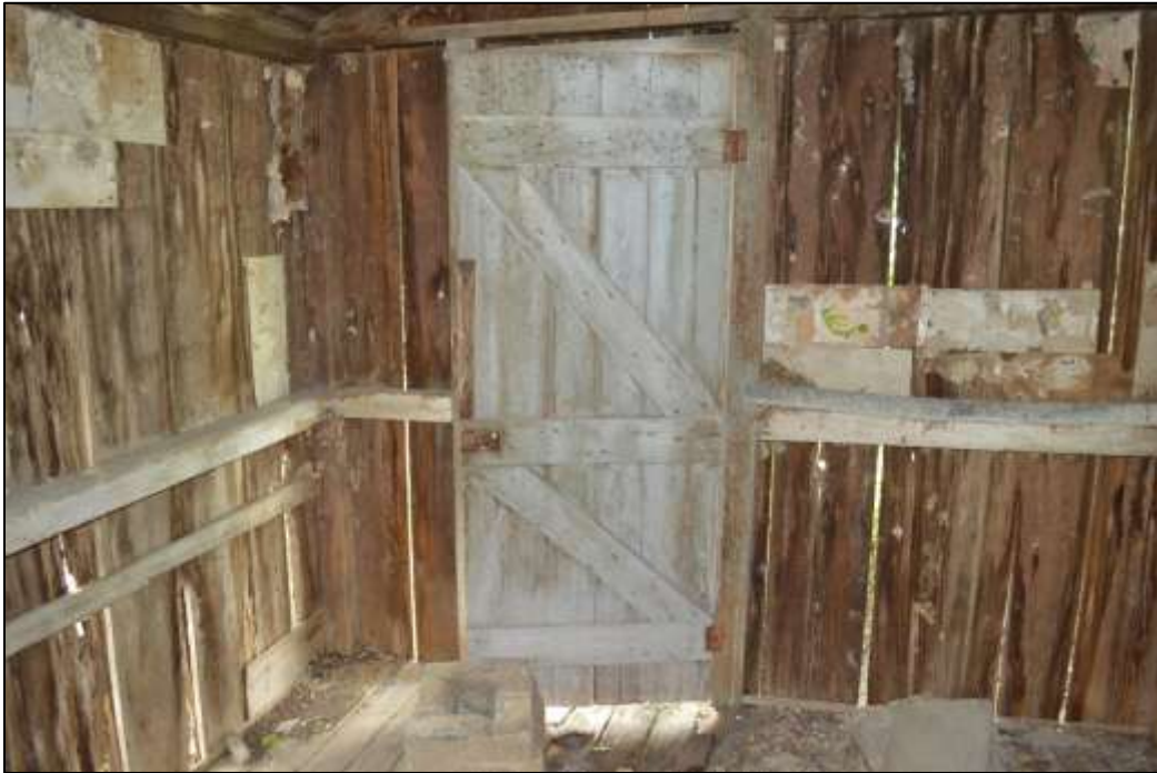
47. Interior kitchen door in NE room
