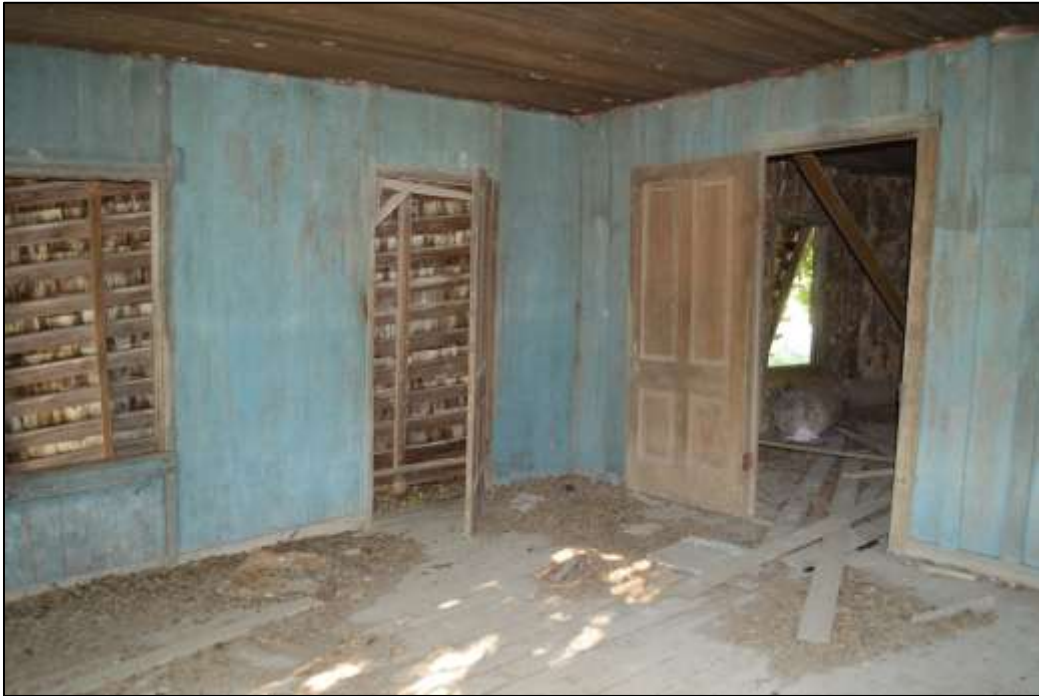
57. Interior overview of southeast room
