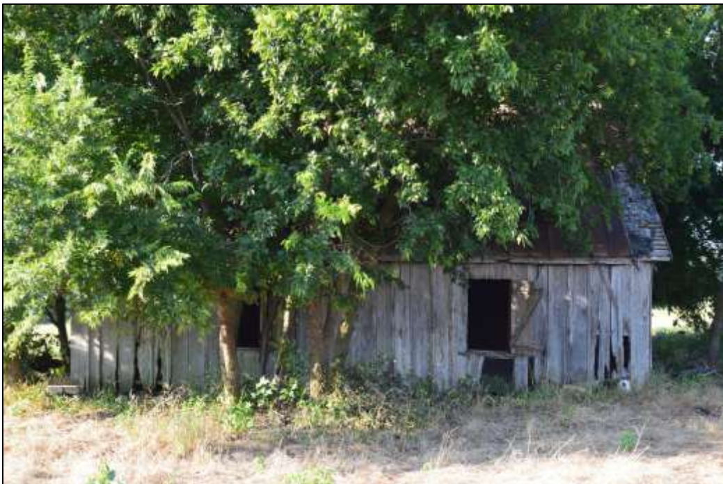
04. North façade of house
