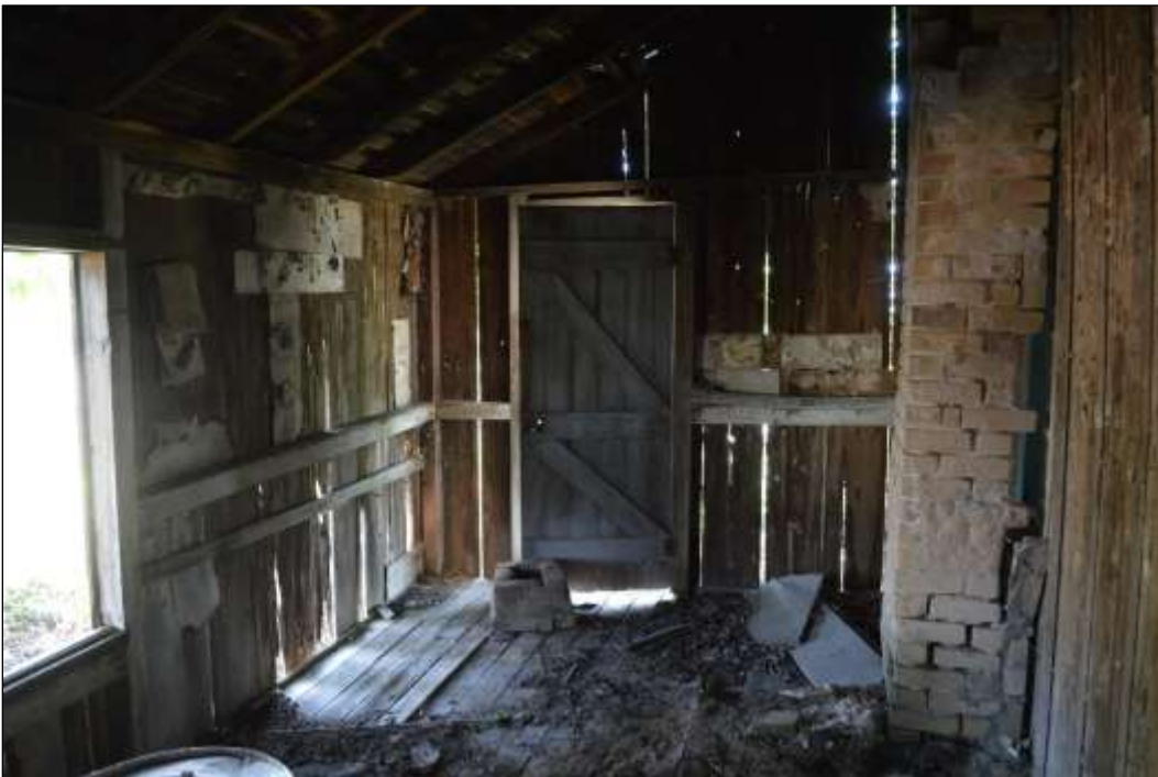
Figure 14. View of Northeastern Room (Note Flue at Right) (Facing East)
