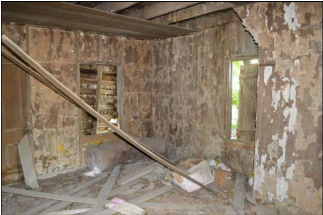
53. Interior overview of southwest room
