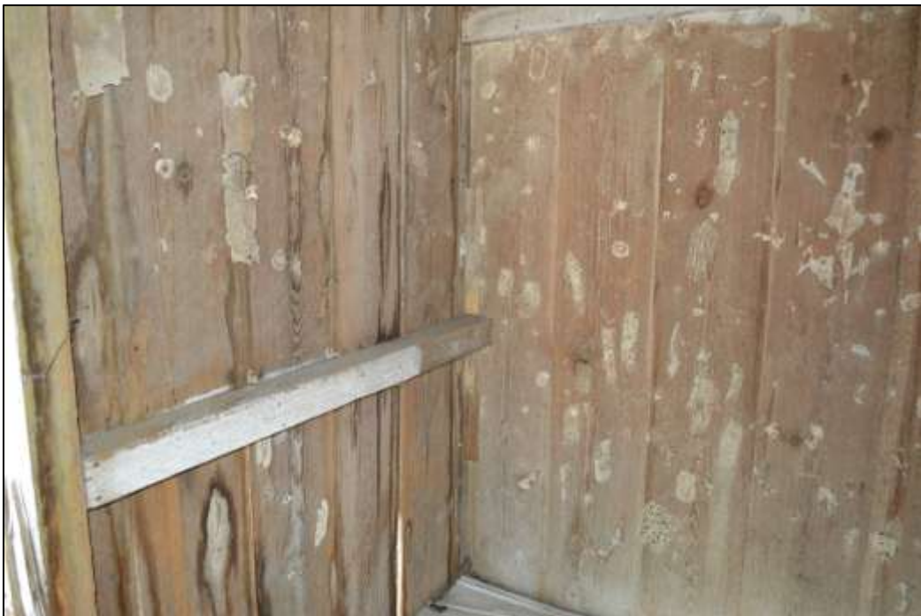
46. Interior walls in northwest room
