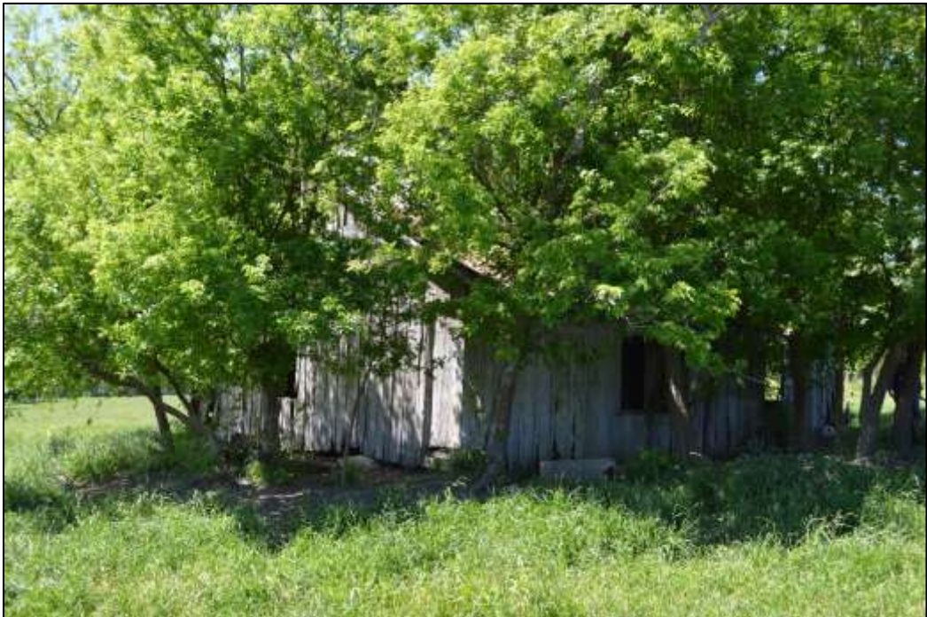
06. North and east façades of house
