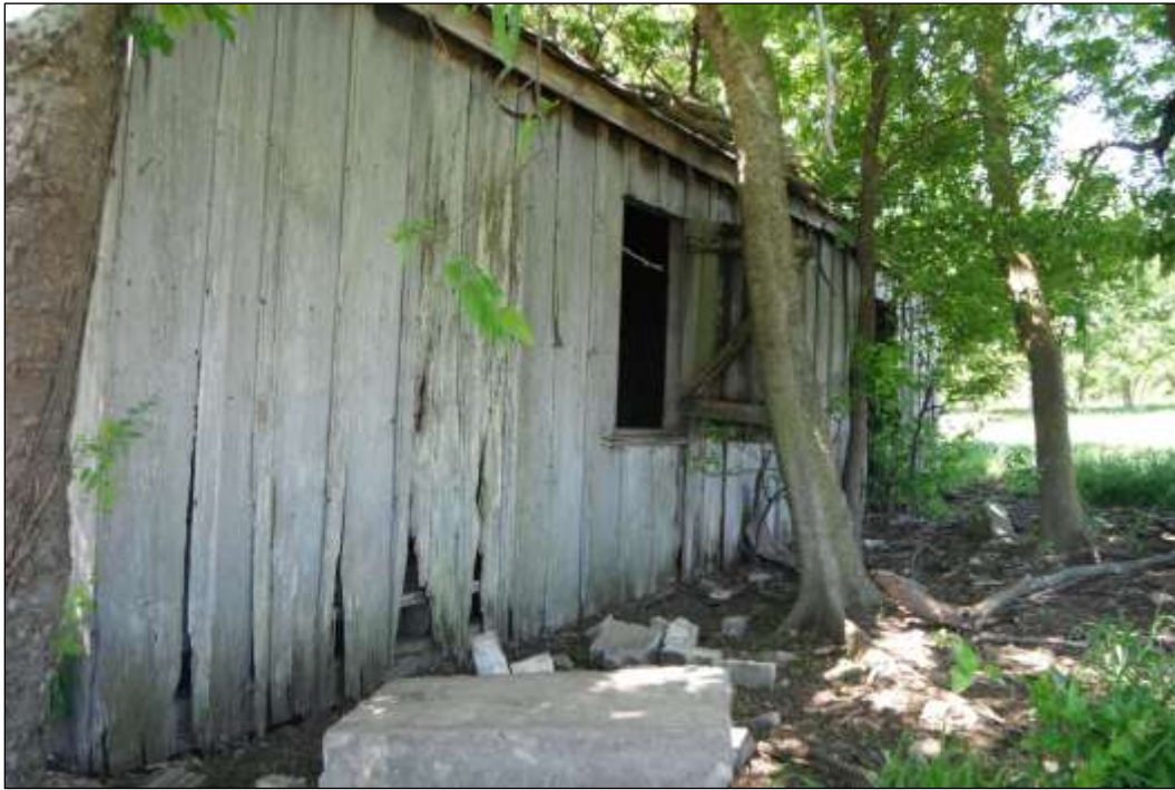
Figure 9. View of Northern (Rear) Façade of House (Facing Southwest)
