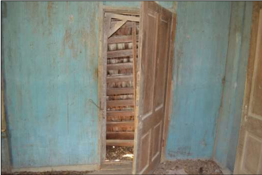
49. Interior walls and door in southeast room
