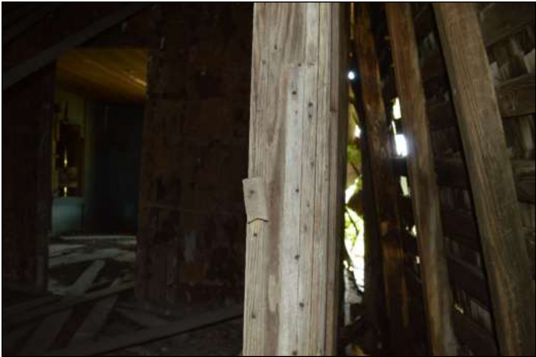
30. Window jambs and rail guards on south façade
