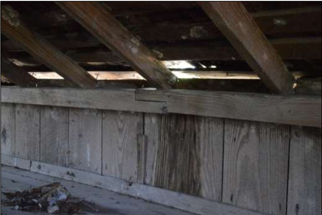
38. Roofing in loft showing lapped plates and rafters
