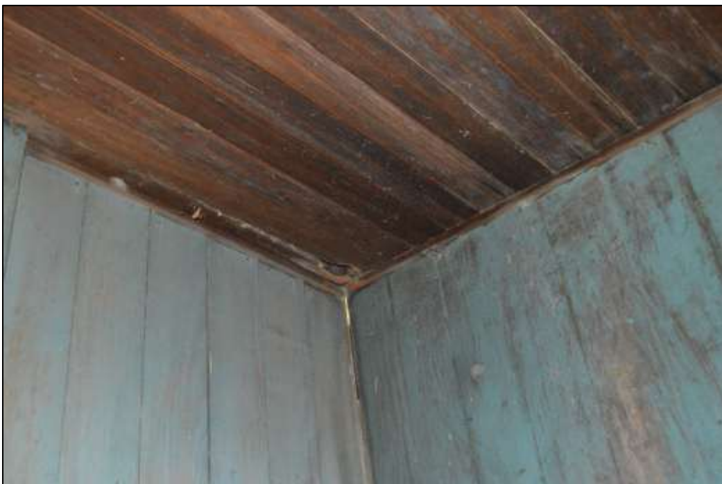
64. Ceiling in southeast room with bead board
