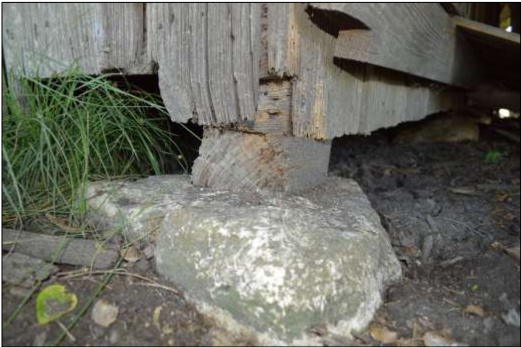
13. Limestone pier supporting southwest corner of foundation
