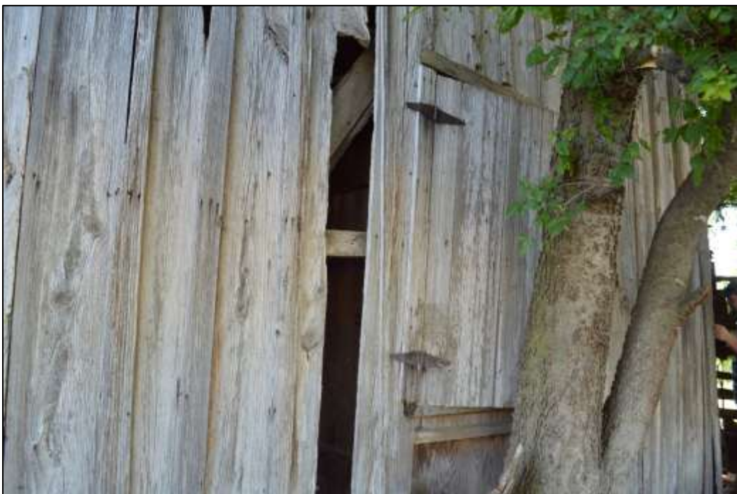
28. Exterior wall and window on west façade
