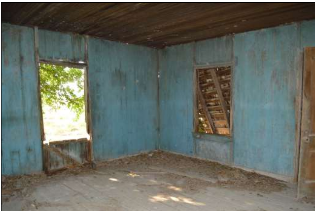
56. Interior overview of southeast room
