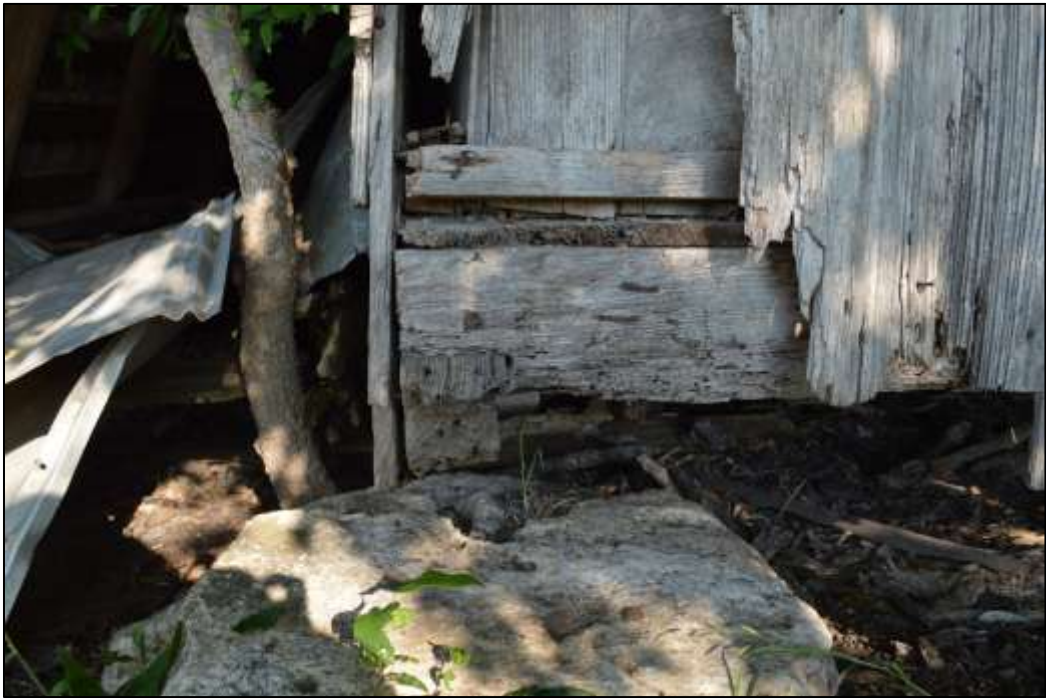
14. Floor construction at southeast corner of house showing floor beam
