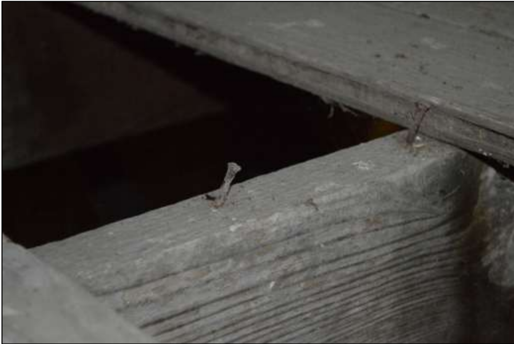
67. Square nails in flooring of loft
