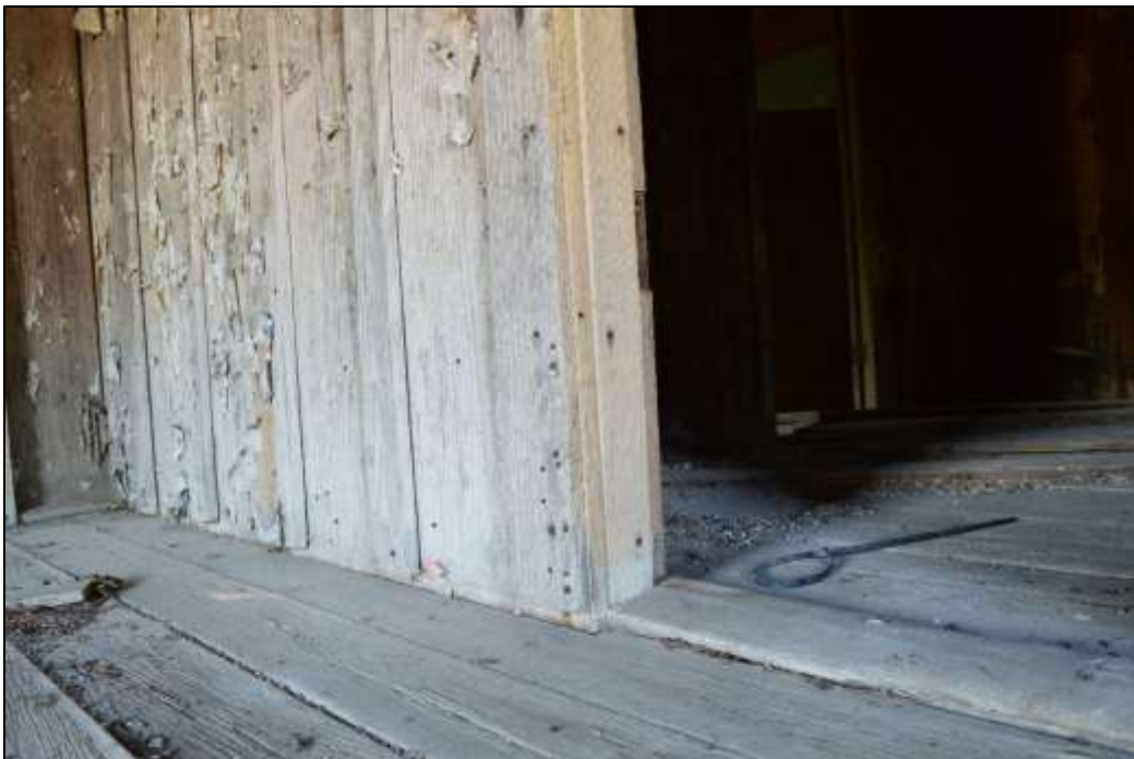
50. Interior flooring and walls in northwest room; note threshold
