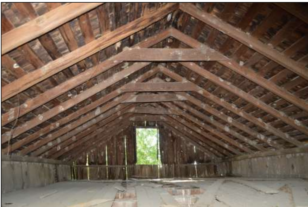
36. Loft level showing rafters, bracing, and floor joists
