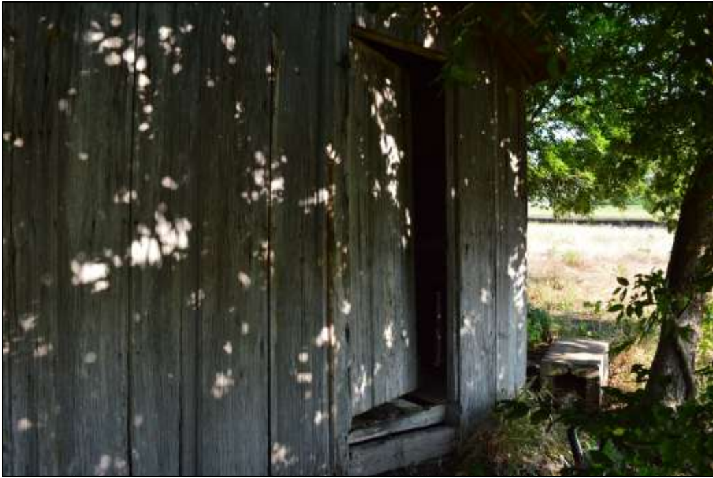
17. Exterior of kitchen door on east façade of house
