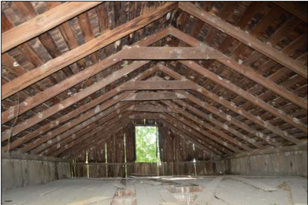
66. Interior of loft
