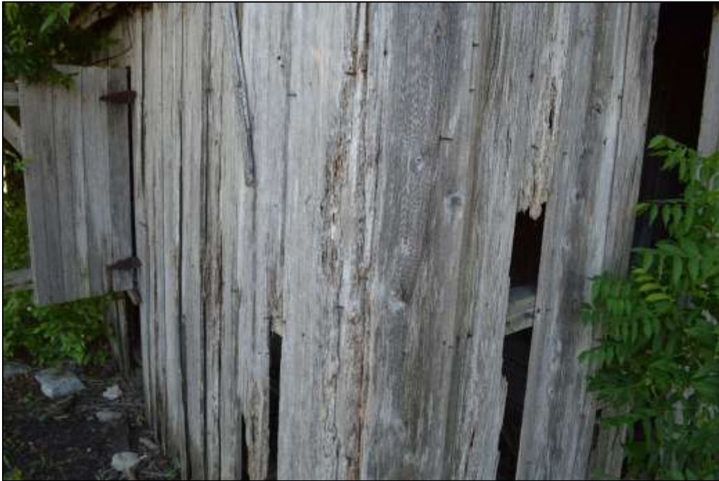
15. Exterior walls at northwest corner of house
