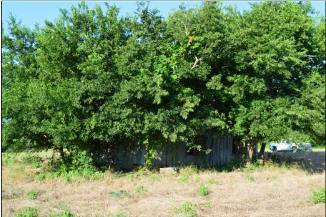
05. North and east façades of house
