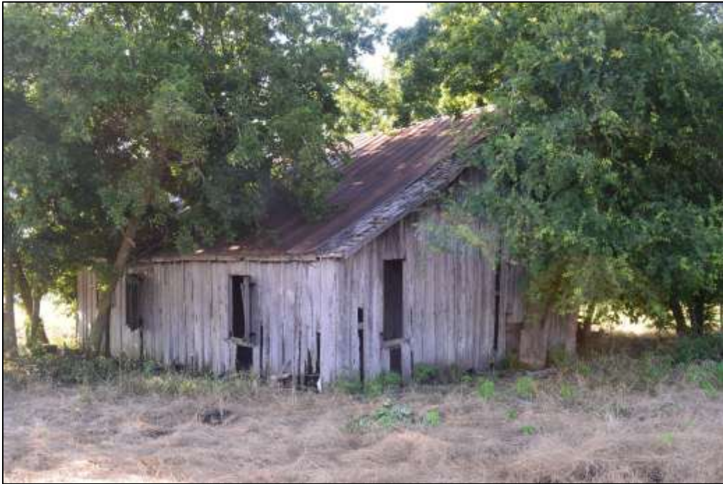
03. West and north façades of house
