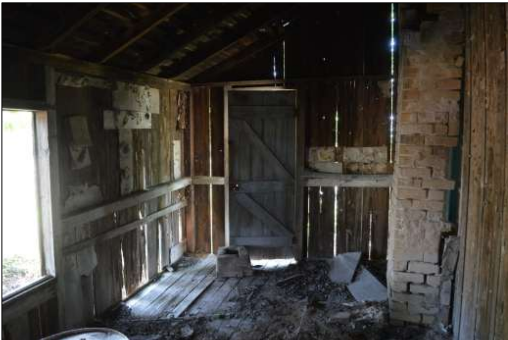
58. Interior overview of northeast room (kitchen)
