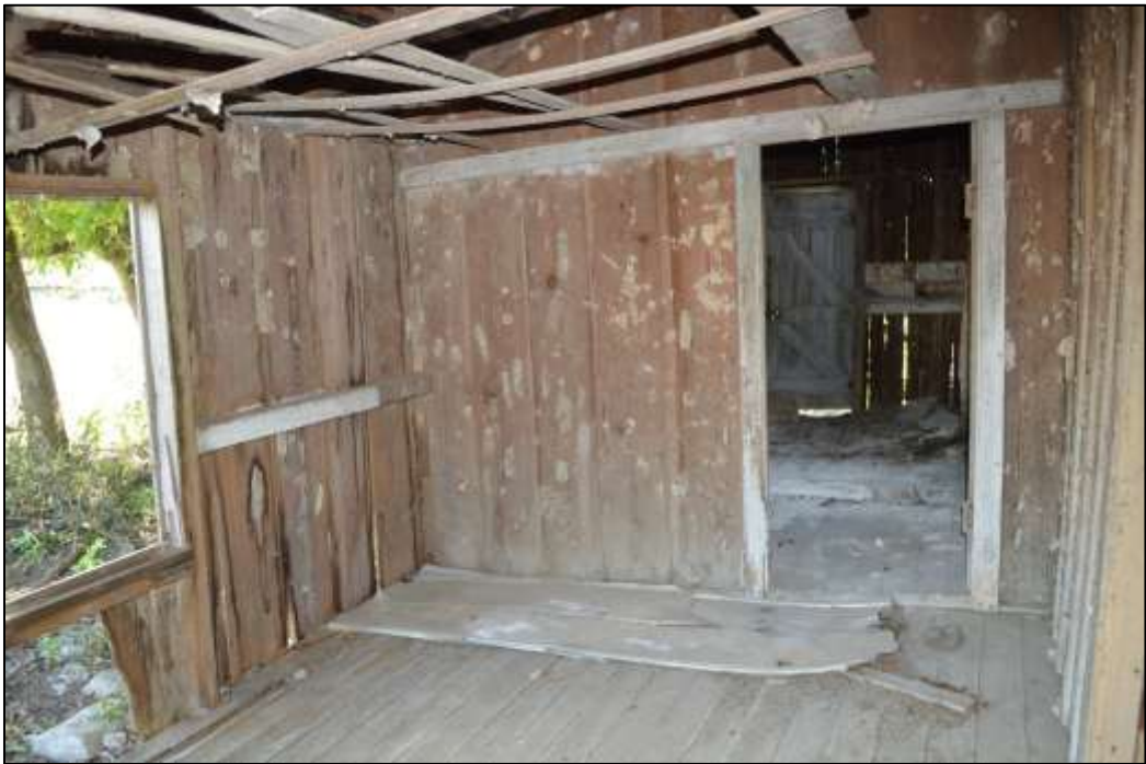
61. Interior overview of northwest room
