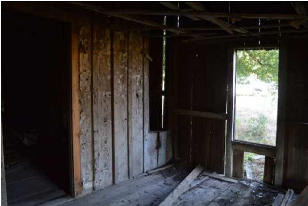
60. Interior overview of northwest room
