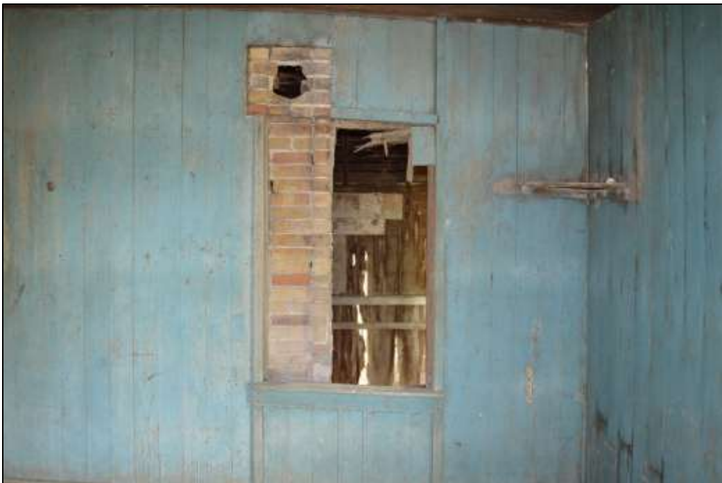
48. Interior walls in southeast room; note stove flue port in chimney
