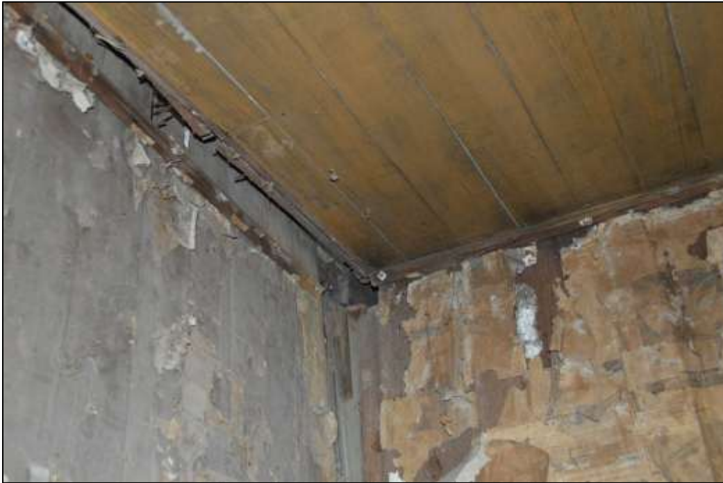
63. Ceiling in southwest room
