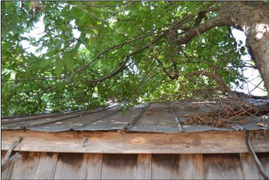
27. Exterior roofing, taken from north façade
