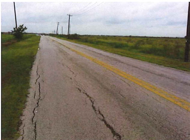
Segment from SH 130 to Weiss Ln – facing west
