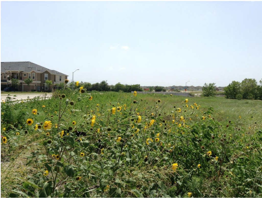
Photo 1: Typical view of project area from the east side, facing west towards the culvert crossing at Town Center Drive.
