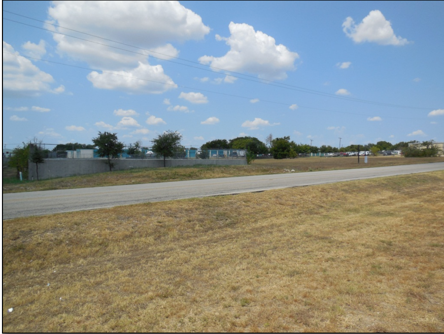
Existing detention pond on the southeast side of the property, as viewed from Old Austin Hutto Road
