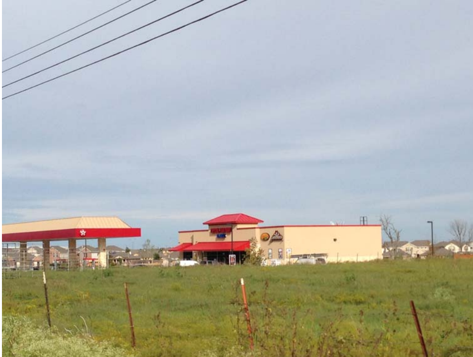
EXISTING GAS STATION - NORTH OF SUBJECT SITE
