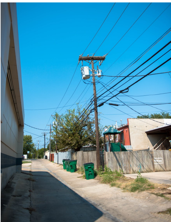
Existing Conditions along Alley
