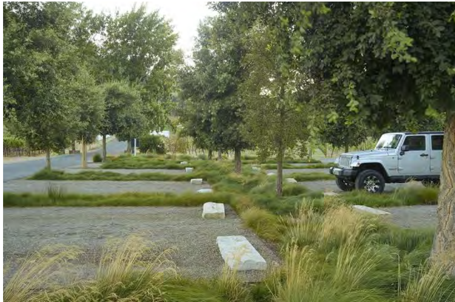
An example of a surface parking lot with pervious pavement system (Odette Winery - Napa, CA).
