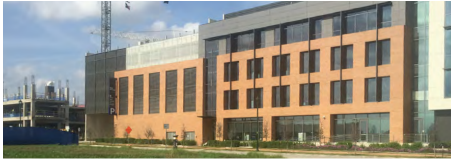
An exposed garage treated with high quality materials and treatments
