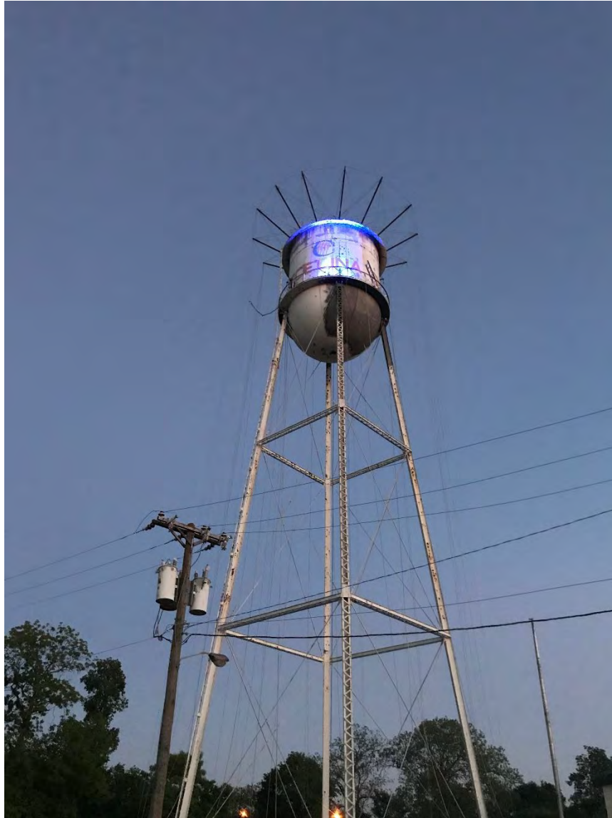
Example Balcony Light Mock-Up Test (Alternate Bid Item #3)
