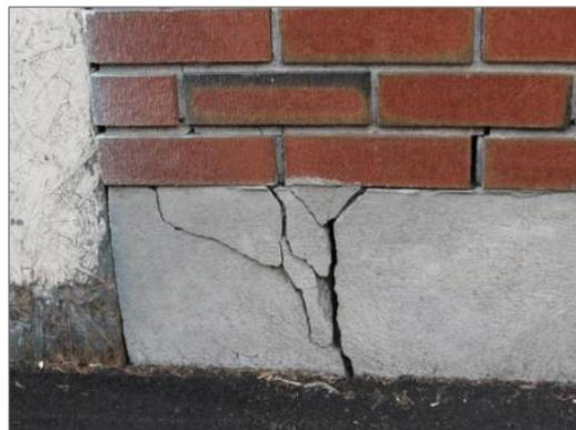
Cracked foundations and floors, jammed windows and doors, and ruptured pipelines are typical types of damage resulting from swelling soils. Damage to the upper floors of larger buildings can occur when motion in the structure is significant. While all infrastructure within the Travis County planning area,
