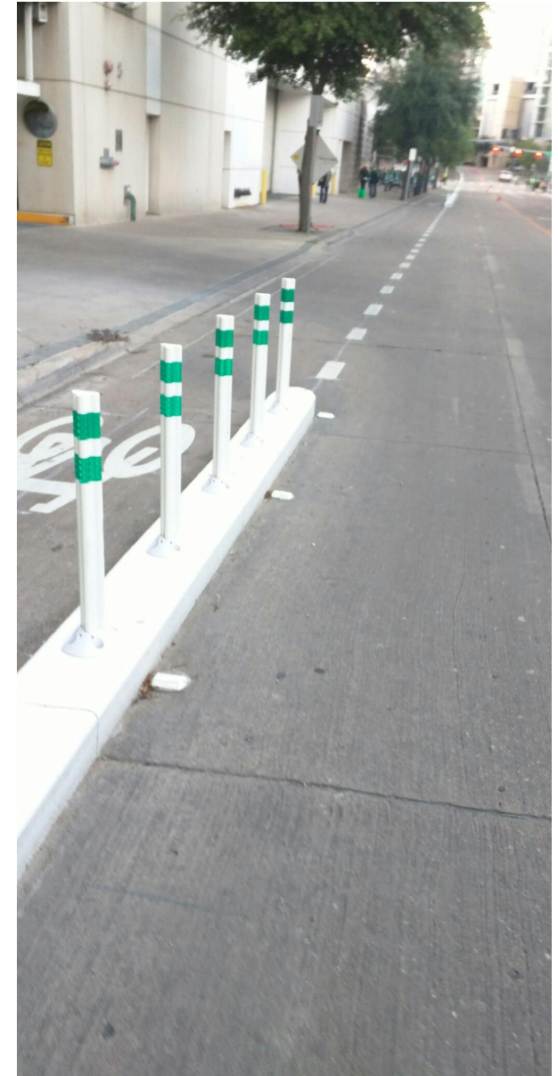
Protected bicycle lane in urban setting
