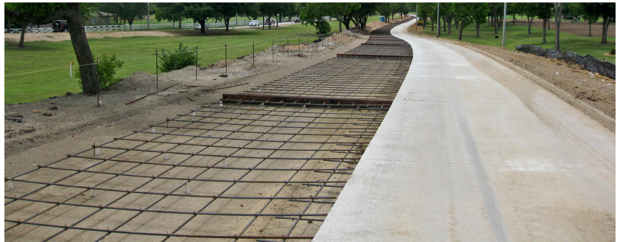
Roadway under construction
