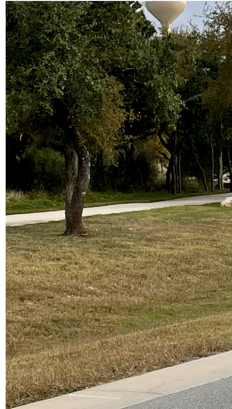
Roadway with ribbon curb, swale and sidewalk/trail
