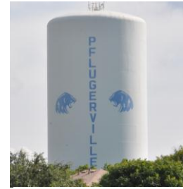
Pflugerville Water Tower
