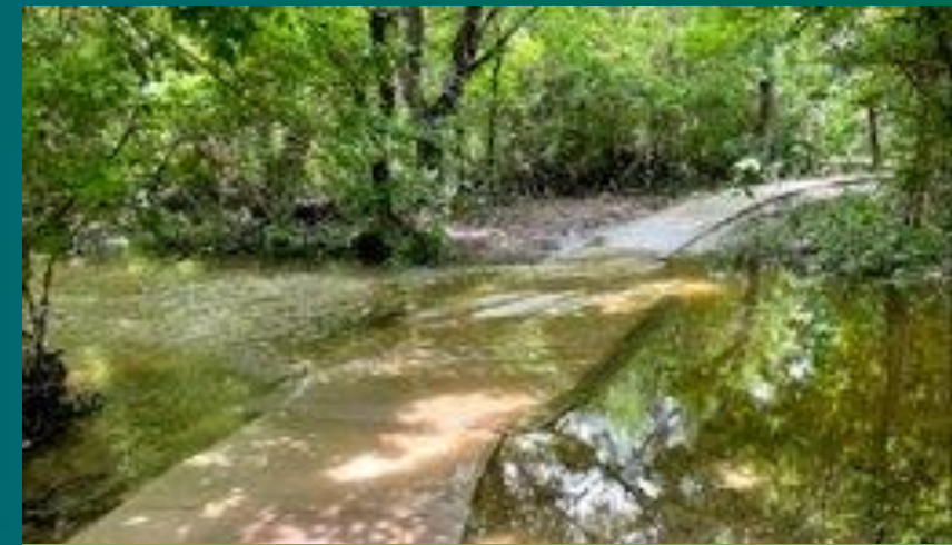
6/1/2021 Project Team Site Visit – Murchison/Mallard Park existing drainage condition
