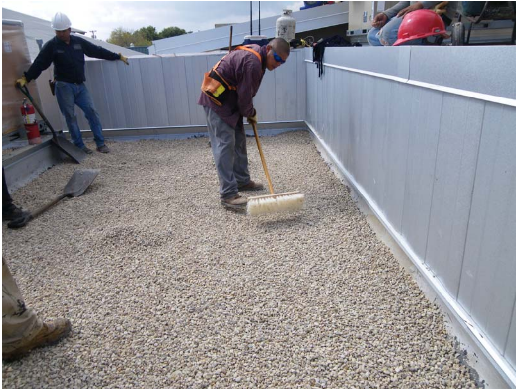
▲ Installing aggregate on the flat roof system.
