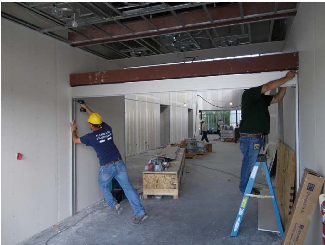
▲ Installing the automatic sliding entrance door system.
