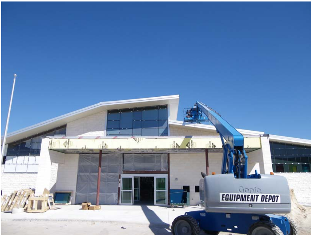
▲ Installing permanent glass on the upper frame systems.
