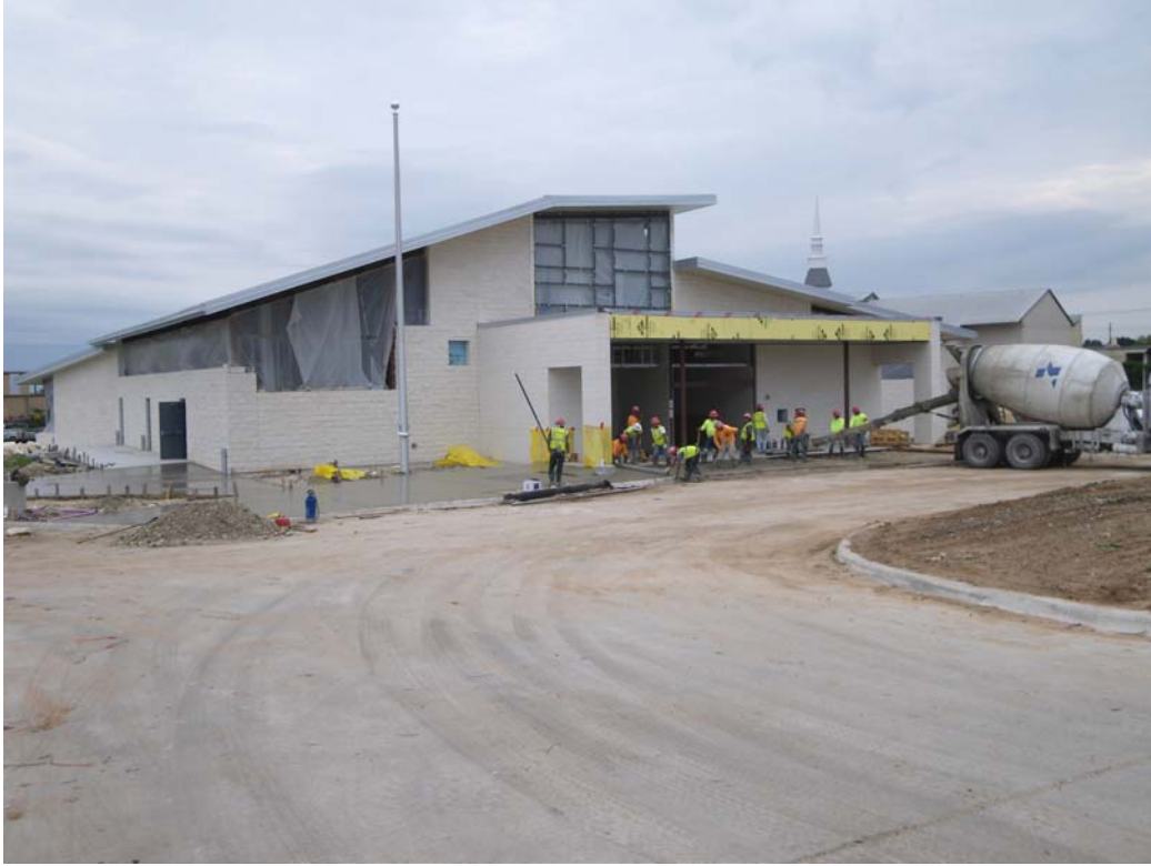
▲ Concrete pour at the main entrance area.
