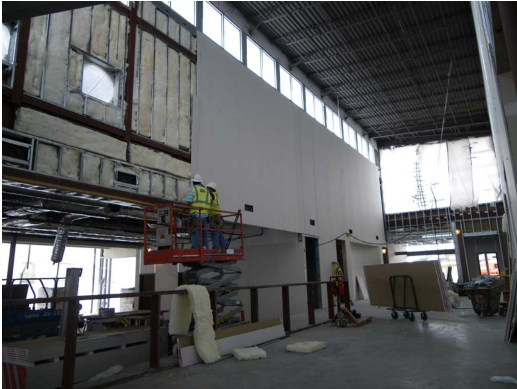
▲ Insulation and drywall placement in the main hallway.
