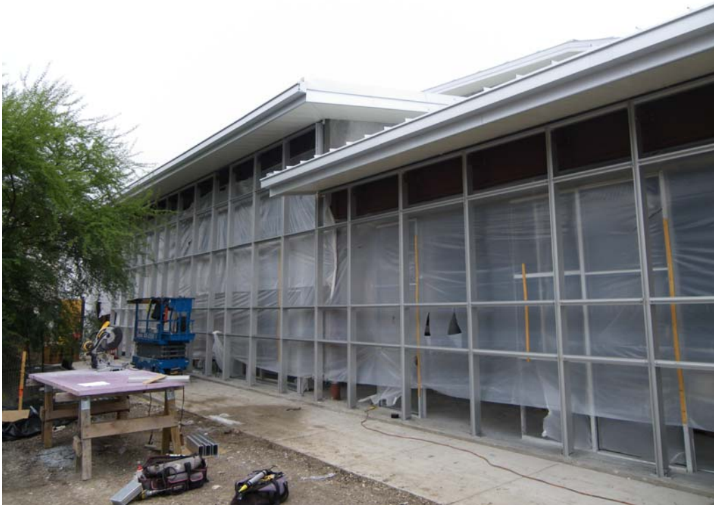
▲ Curtain wall framework installation on the north face of the library.
