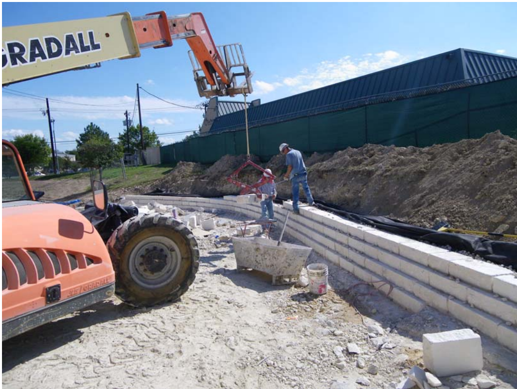
▲ Constructing the courtyard retaining wall.
