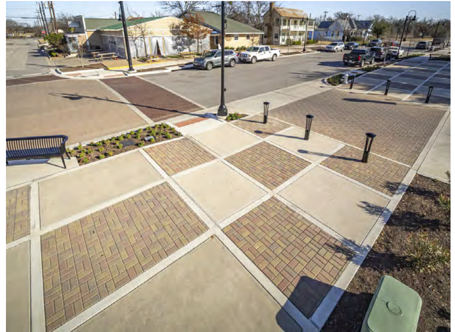
Pavers intermixed with concrete pavement.
