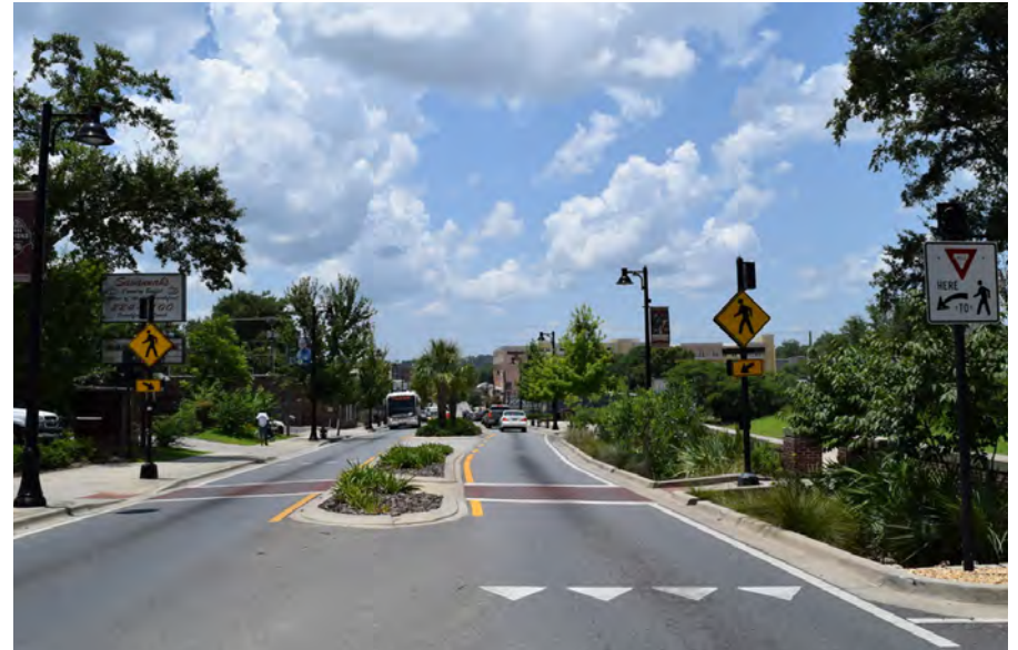
Vehicular point of view of a pedestrian island.
