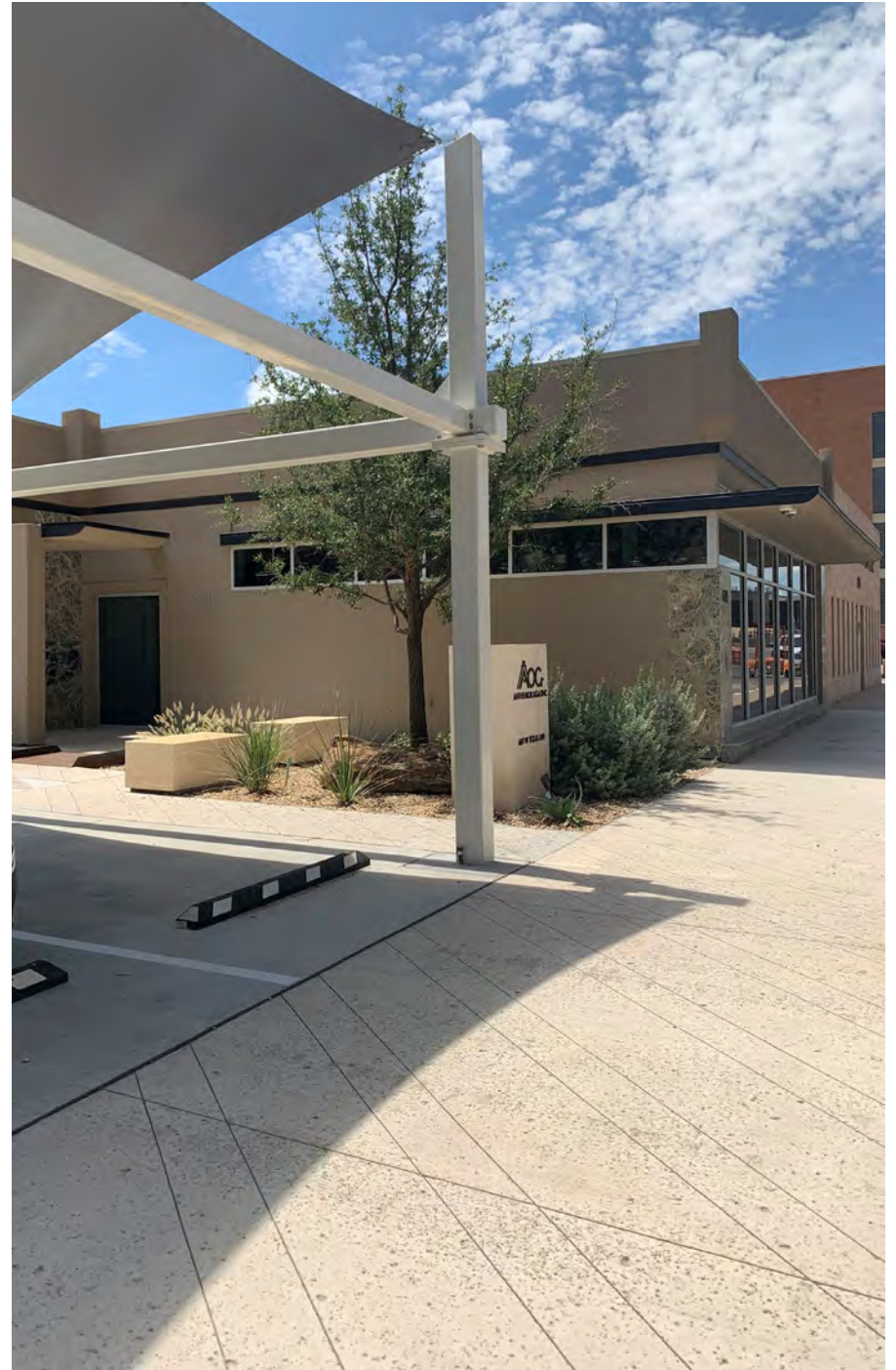
This concrete sidewalk has been treated with rock salt and control joints.
