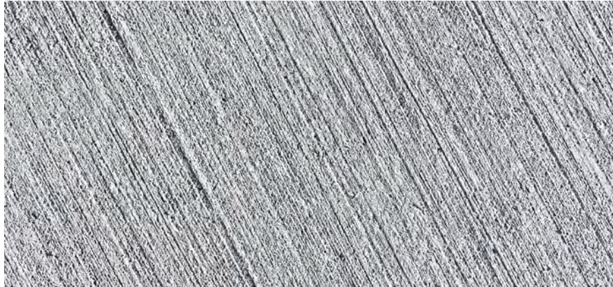
Broom finish concrete
