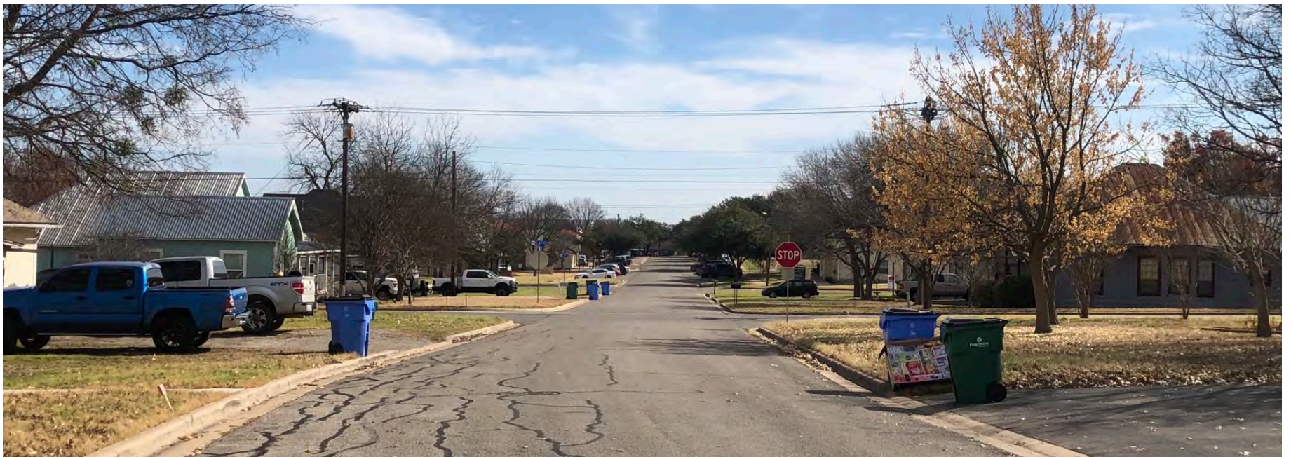
West Main Street viewing toward 4th Street.
