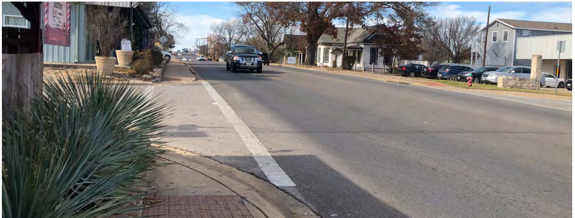
Narrow sidewalks that are directly adjacent to curbs in Section Two do not encourage pedestrian activity.
