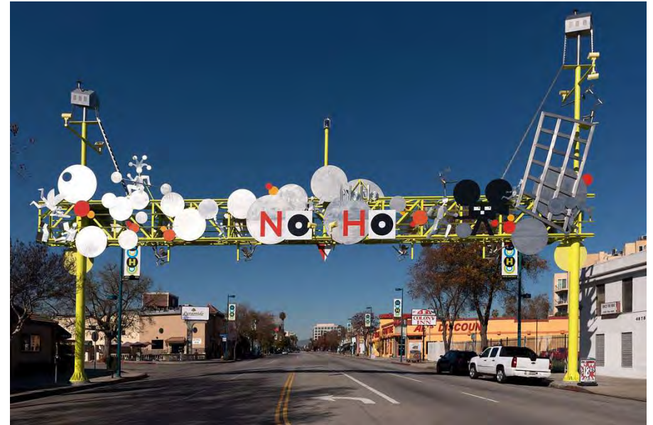
Overhead gateway signs can span across the entire roadway.
