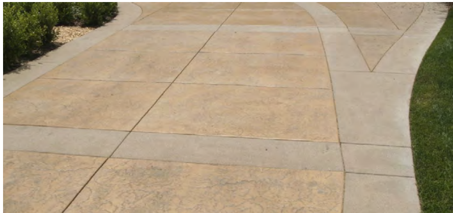
Integral colored concrete with control joints
