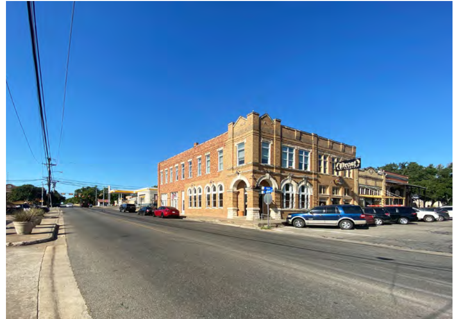
Existing view from northeast corner of Main Street and Railroad Avenue.
