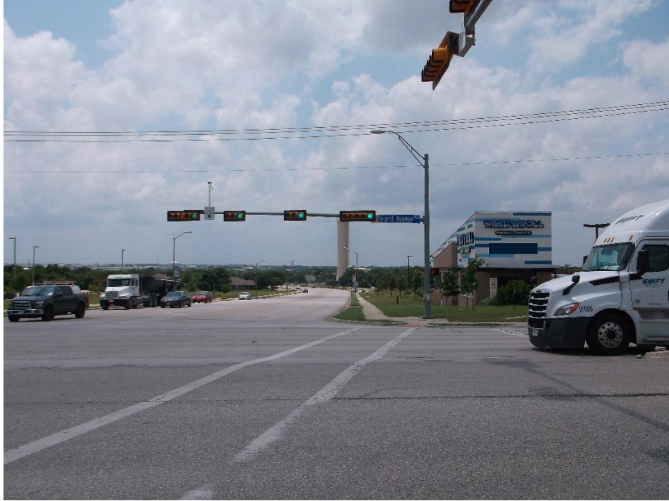
WB approach on FM 1825. Needs 4-section Flashing Yellow Arrow left-turn signal.
