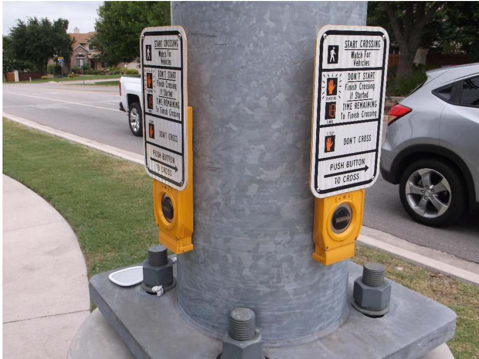
NW corner pedestrian push buttons
