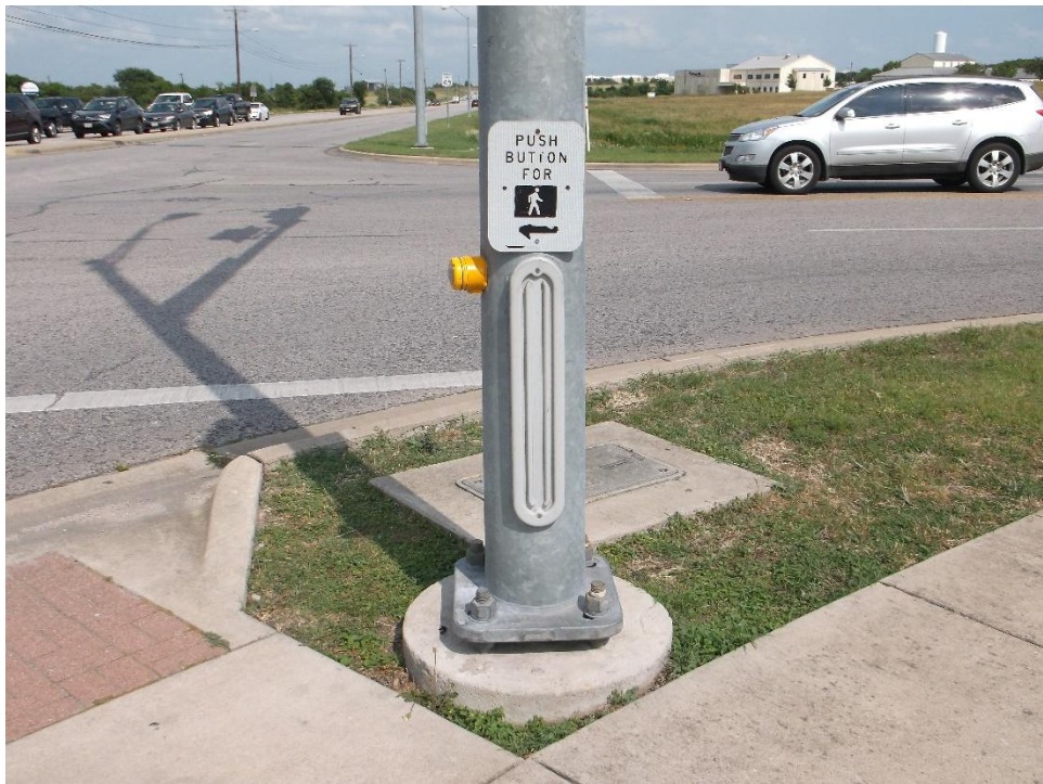
Pedestrian push button on SW corner does not work
