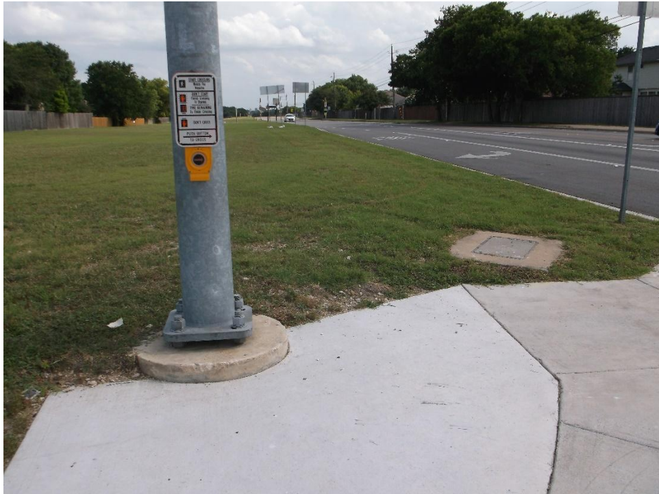
Pedestrian push button on SE corner is too far from ramp
