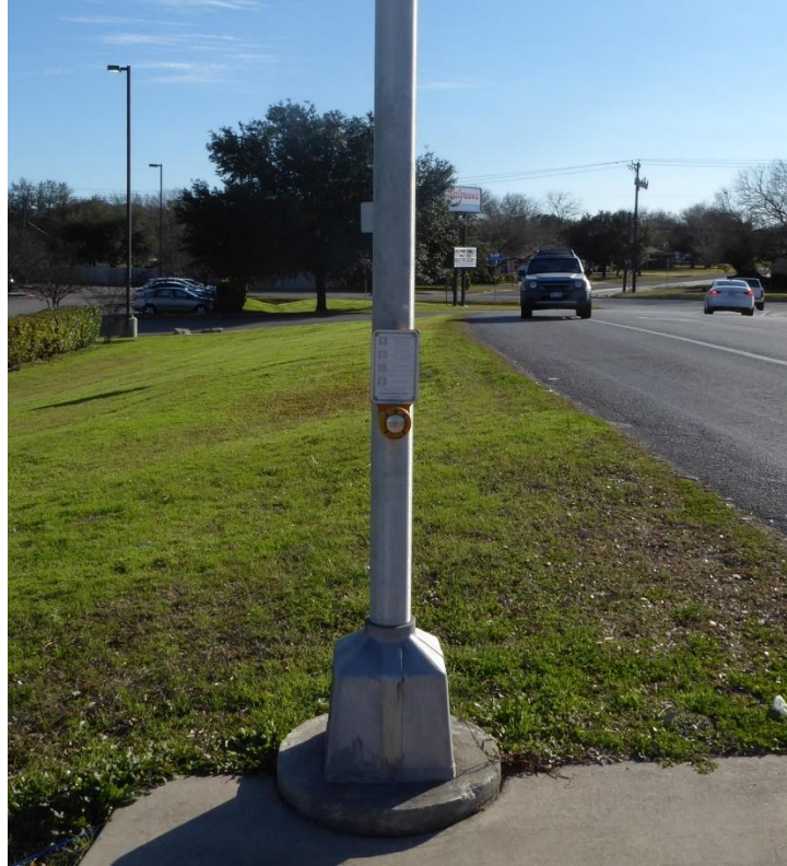
SE corner - faded pedestrian crossing sign and push button not working
