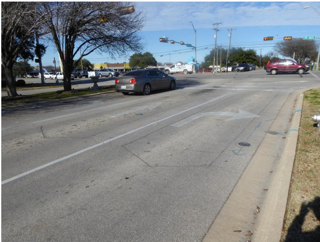
Loops located on NB approach on Central Commerce
