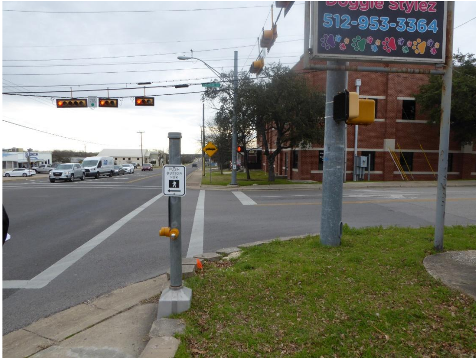
Pedestrian push button on separate pole of pedestrian head
