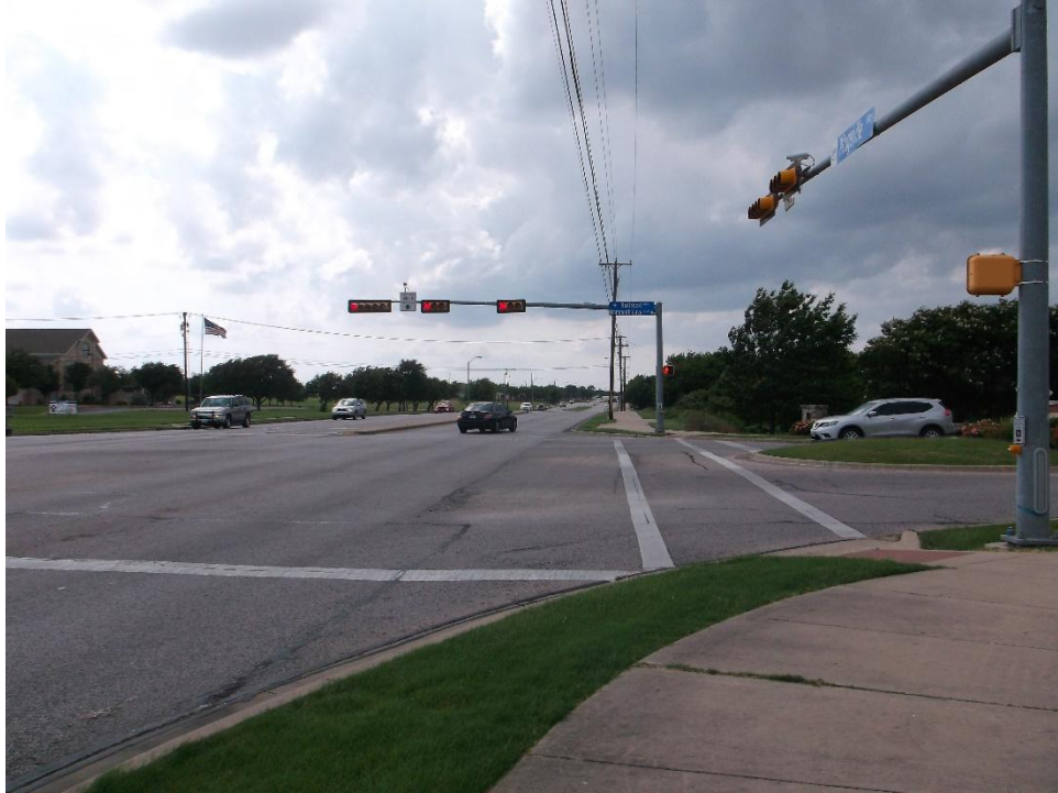
WB approach on Pflugerville Parkway. Needs 4-section Flashing Yellow Arrow left-turn signal.
