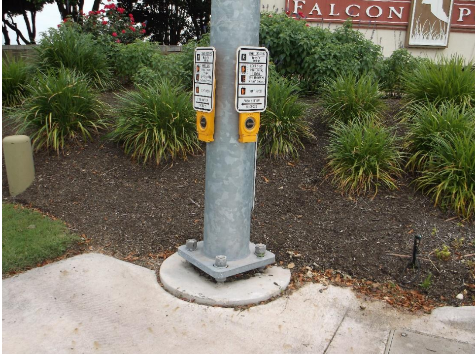
Pedestrian push buttons at SE corner
