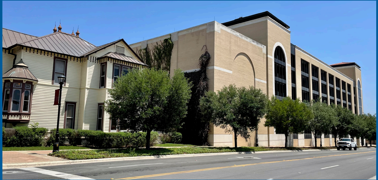
A parking garage in the region
