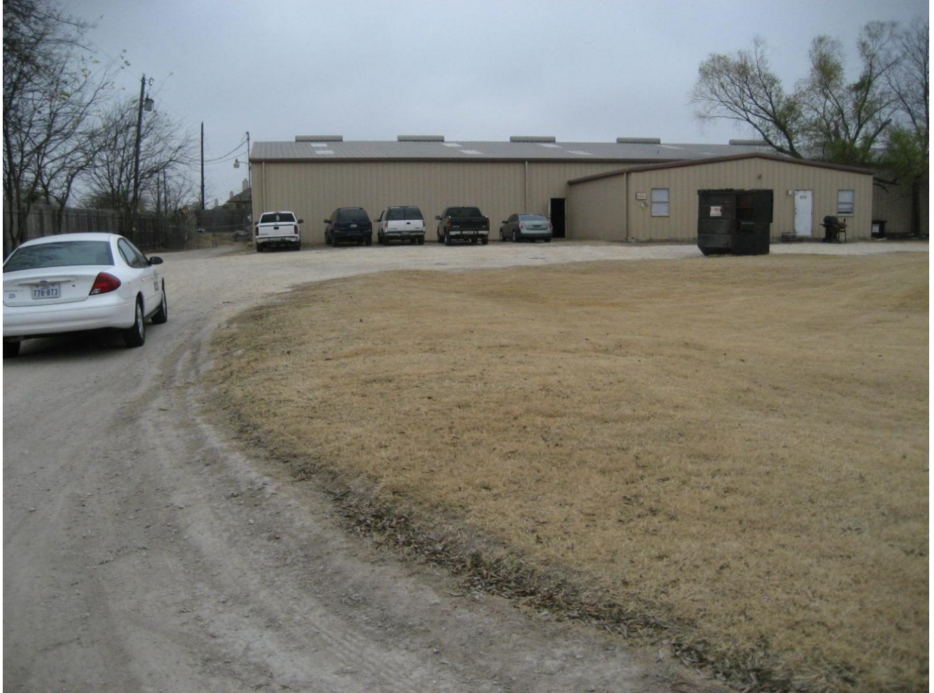
Facing South on Kelly Lane (Subject Site)
