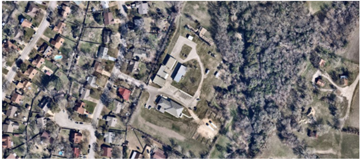
PAWS facility is shown to the east of the neighborhood
