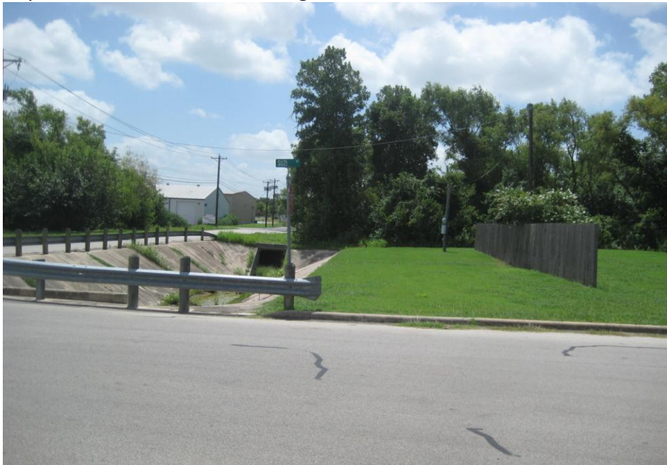
Royston Lane at Suzi Lane looking east:
