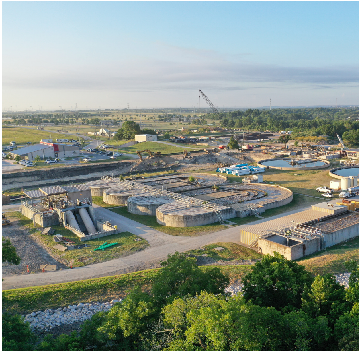
Wastewater Treatment Facility
