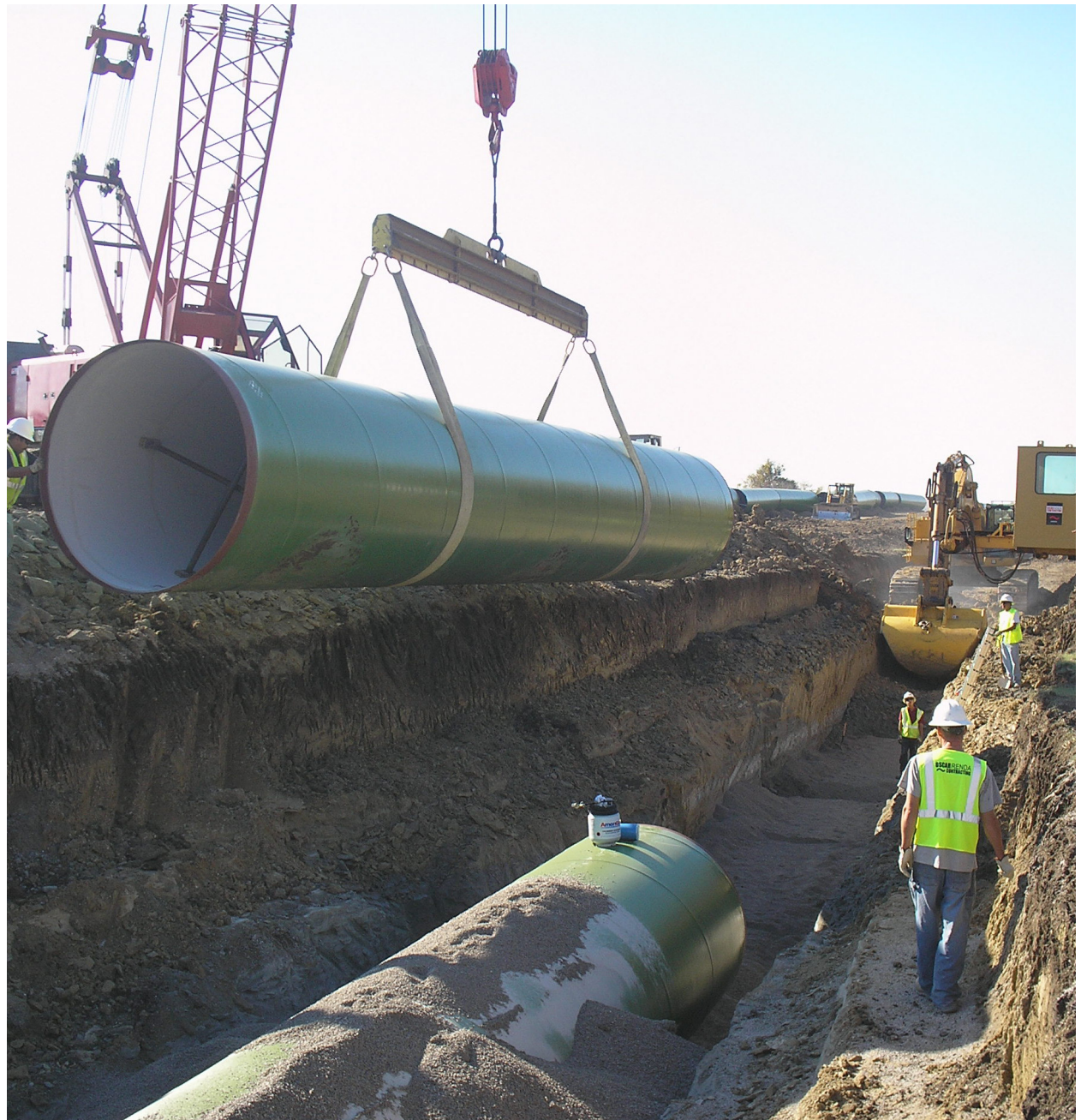
Utility line installation
