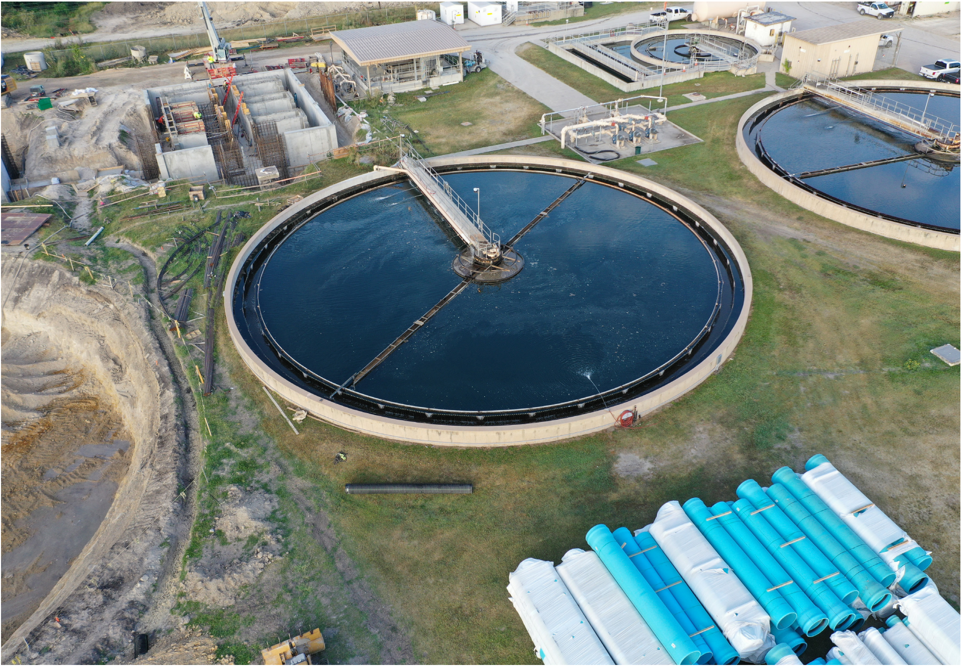
Pflugerville Central Wastewater Treatment Plant undergoing expansion
