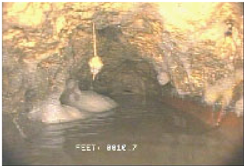
Grease on walls of a sewer pipe
