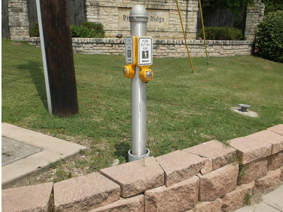
All pedestrian push buttons, including this one on the NE corner, are too far from the pedestrian ramps
