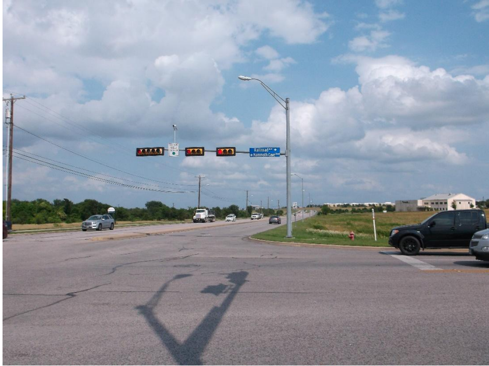
EB approach on Pflugerville Parkway. Needs 4-section Flashing Yellow Arrow left-turn signal.
