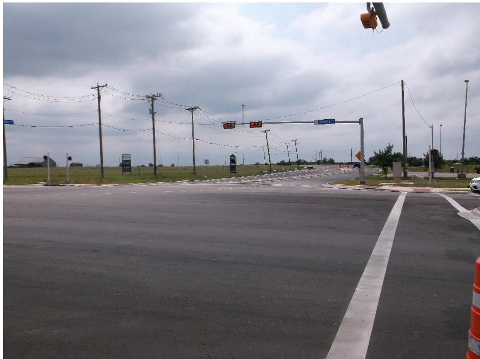
WB approach on Pflugerville Parkway
