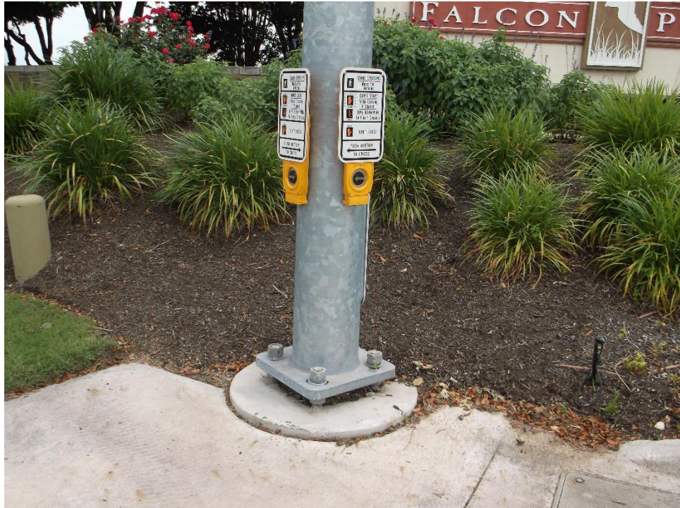
Pedestrian push buttons at SE corner
