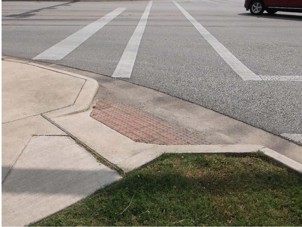
Pedestrian ramp on SW corner (typ.) – ramp aligns toward intersection rather than crosswalk
