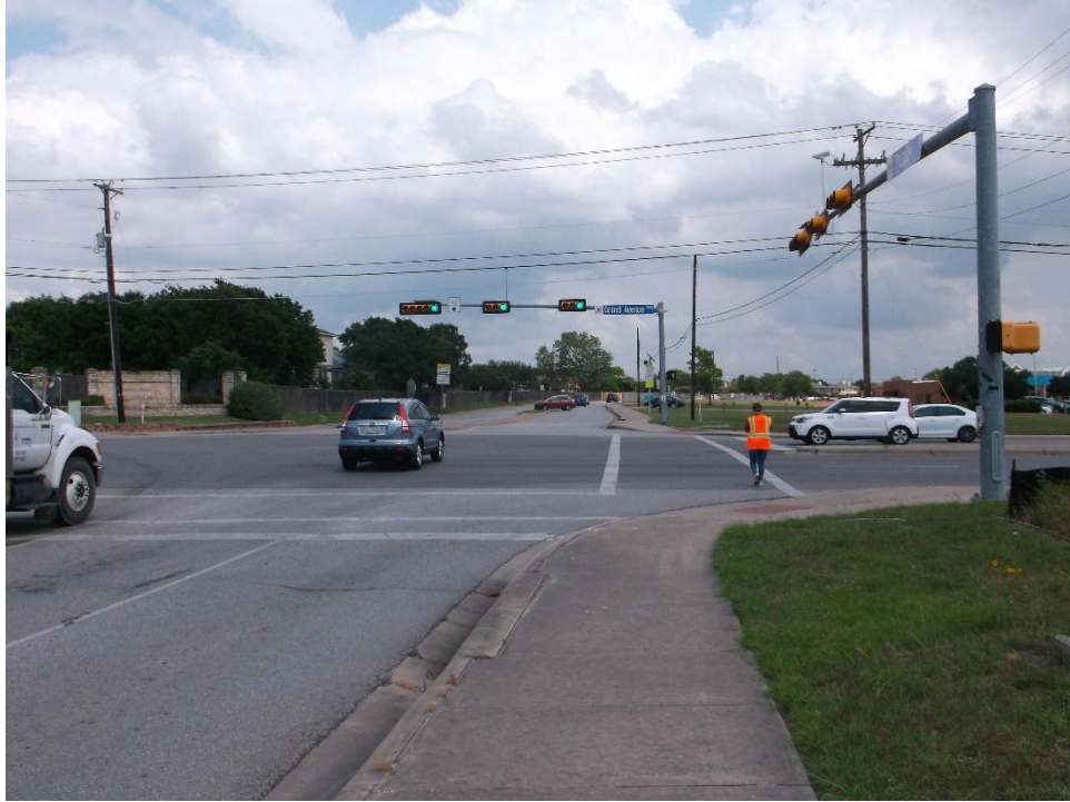
EB approach on Picadilly. Needs 4-section Flashing Yellow Arrow left-turn signal.
