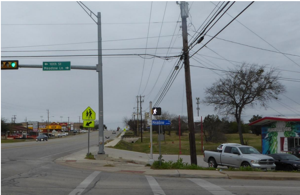
SE Corner – relocate ped push-button to align with south crosswalk and accessible ramp
