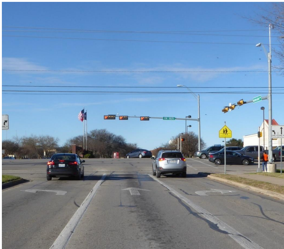
Mast arm pole on NE corner – provide min. 8' center to center spacing between signal heads
