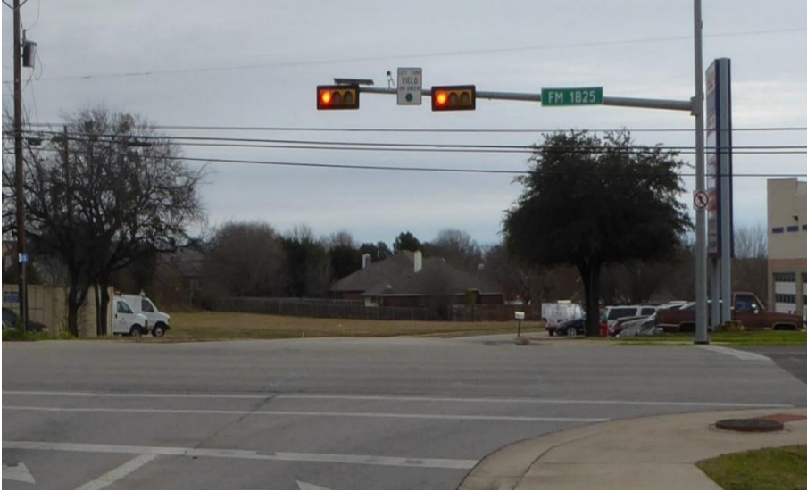
Split phase on NB approach on Meadow Ln
