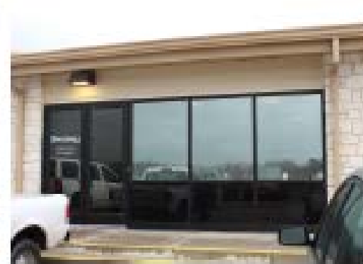
Public Works Facilities 15500 Sun Light Near Way 2,668 sf (CIP staff space only)
