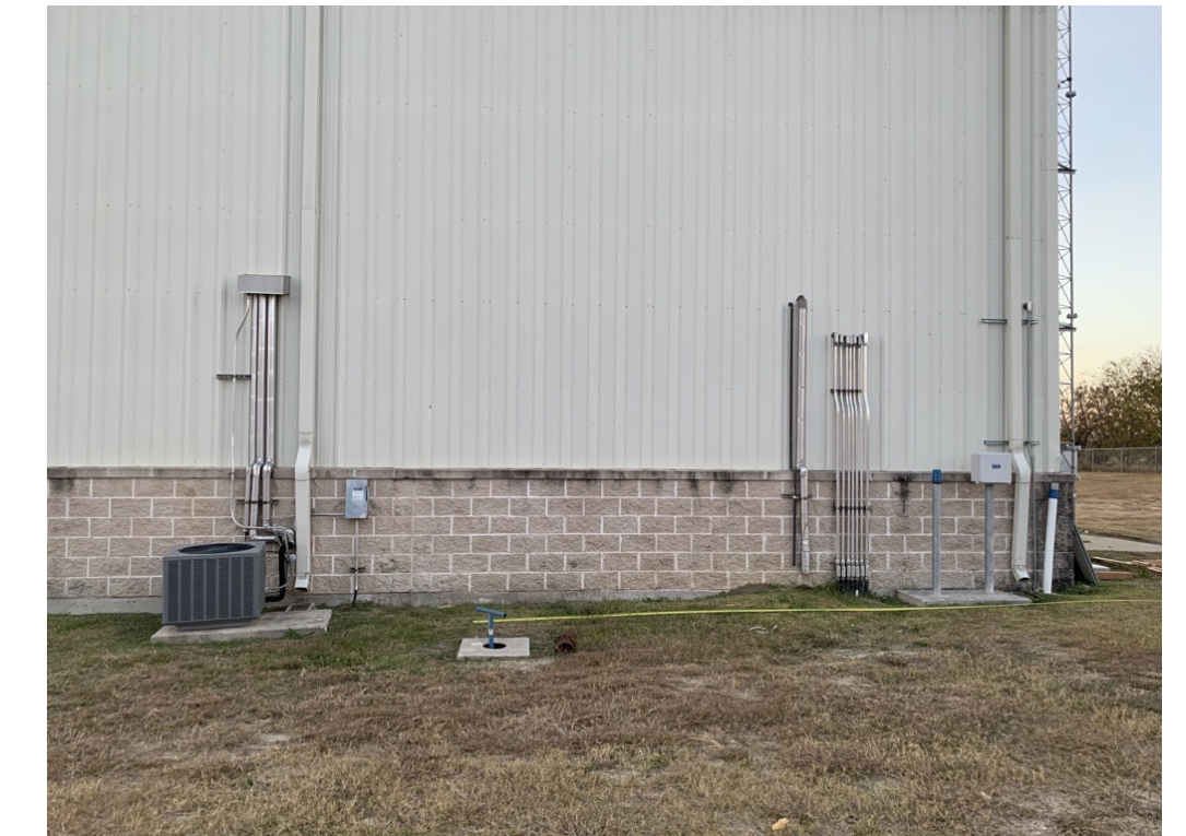
HSPS EAST EXTERIOR WALL
