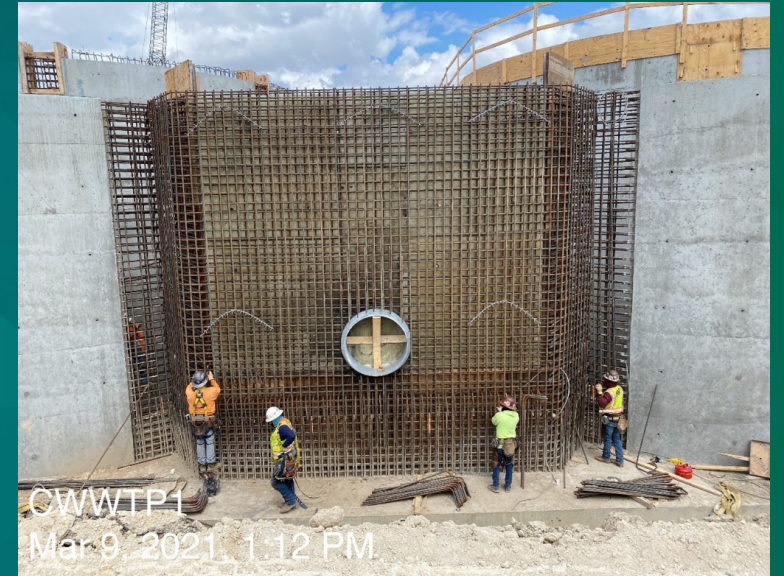
BNR Basin - South End - Effluent Pipe Outlet
