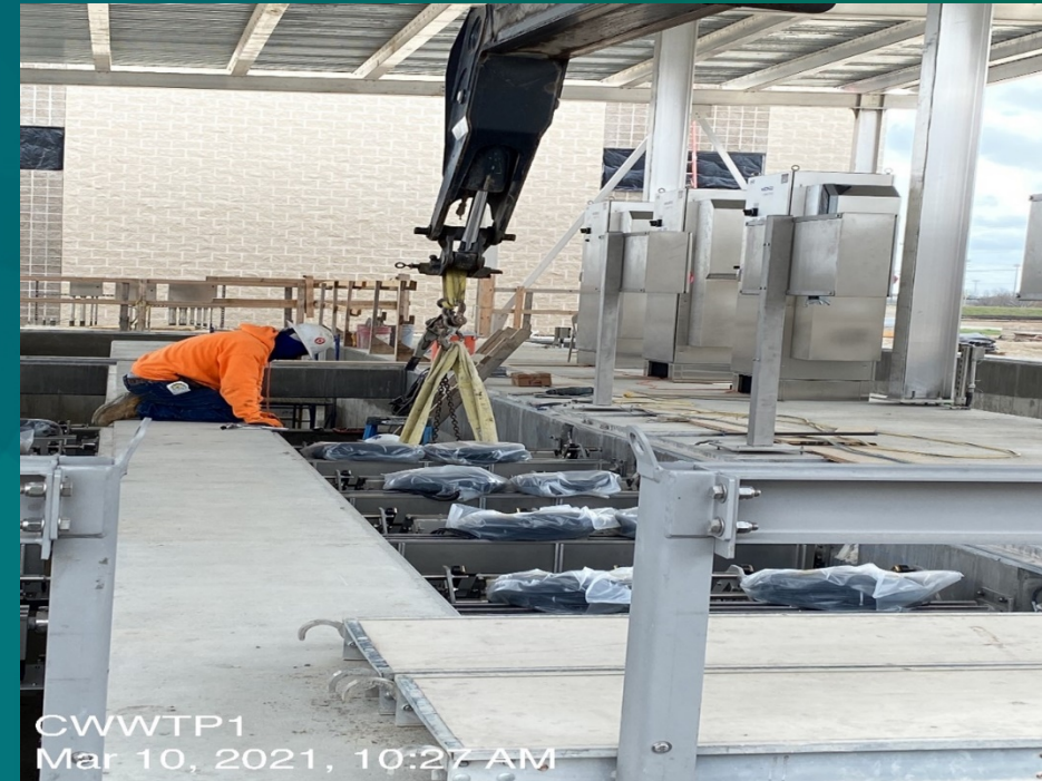
Ultraviolet Basin – Installation of Wiper/Lifting Mechanical
