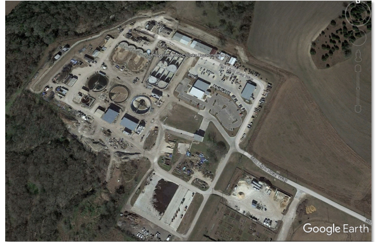
Central Wastewater Treatment Plant
