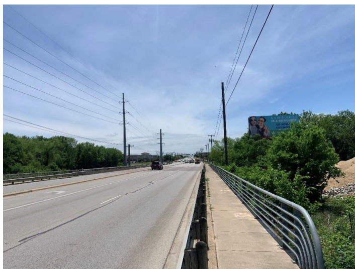
Figure 3-4: Bridge Crossing Wilbarger Creek
