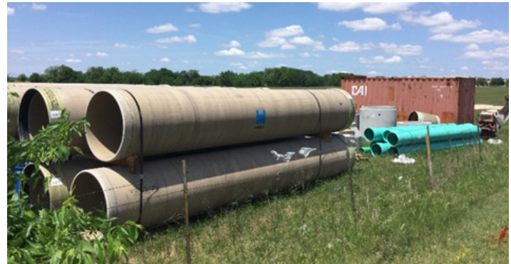
Figure 3-18: Drainage Culverts Prepared for Installation Along FM 685
