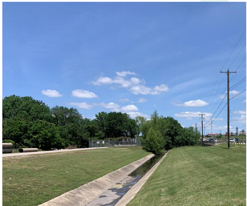
Figure 3-16: Wastewater Lift Station Along FM 685
