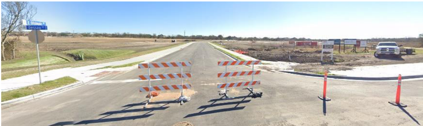
Figure 3-9: Olympic Drive Extension and Brio Apartments
