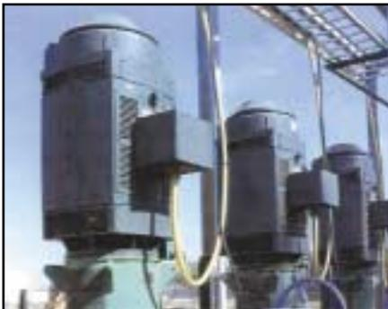
*A clear water feed pump in a paper processing operation is driven by a Weather-Protected NEMA type 1 Duty Master Vertical Motor.*
